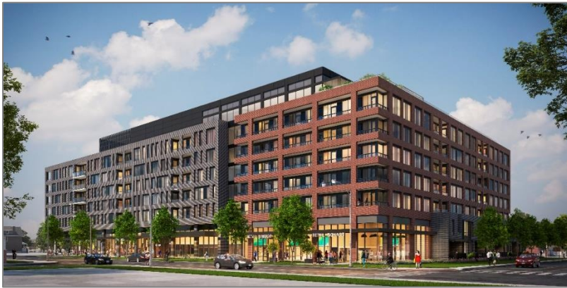
LIUNA/ Fengate mixed use development at 500 Upper Wellington includes geothermal heating/cooling
