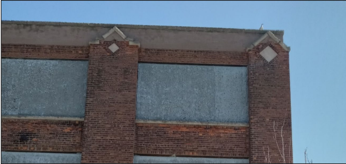
Figure 4: Detail view of decorative elements along roofline of 11 Kelly Street (Structure 3).
