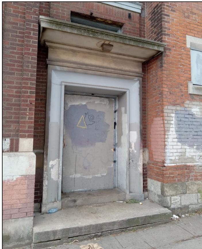
Figure 16: Detail view of the entrance at 134 Cannon Street East (Structure 5).
