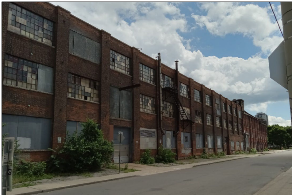
Figure 12: West elevation of the property looking south along Mary Street, including 140-146 Mary Street (Structure 4, left), 130 Mary Street (Structure 1, middle right) and 122 Mary Street (Structure 2, far right).
