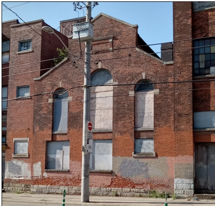
Figure 8: View of the north façade of the eastern portion of 140-146 Mary Street (Structure 4) facing onto Cannon Street East, built circa 1927.
