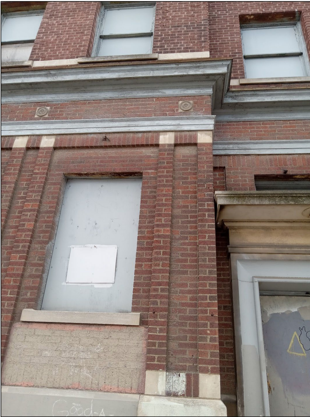
Figure 17: Detail view of decorative elements at 134 Cannon Street East (Structure 5).
