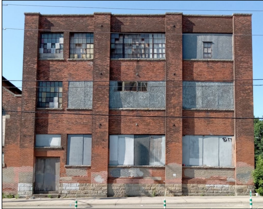
Figure 7: View of the north façade of the western portion of 140-146 Mary Street (Structure 4) facing onto Cannon Street East.
