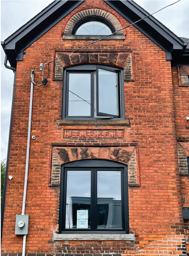
Figure 16. Primary (east) elevation of the residential building located at 89 Catharine Street North showing the windows and rectilinear hood moulds. Page 22
