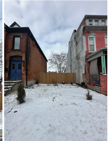
Figure 9. Partial east elevations of 85 Catharine Street North (left) and 89 Catharine Street North (right), showing the gap created by the removal of fire-damaged 87 Catharine Street North.
