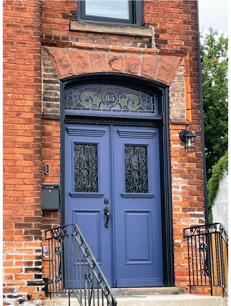
Figure 17. Primary (east) elevation of the residential building located at 89 Catharine Street North showing the door with decorative ironwork and a stained glass transom.
