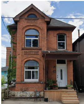
Figure 28. 148 Catharine Street North (Google Maps, 2022).
