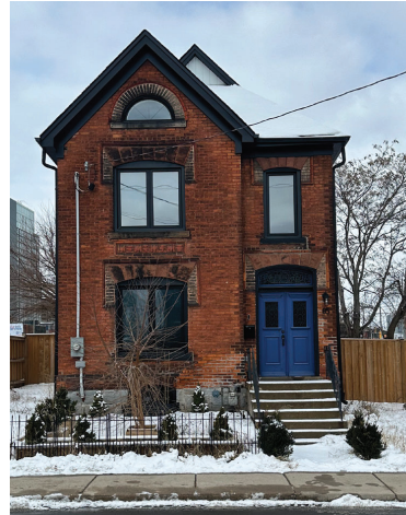
Figure 8. Primary (east) elevation of the property, showing mid and high-rise buildings to the southwest of the Property.
