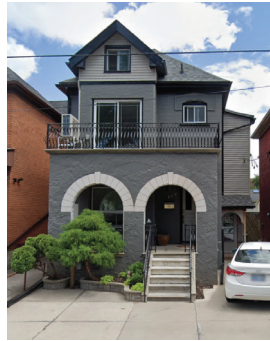
Figure 27. 146 Catharine Street North (Google Maps, 2022).
