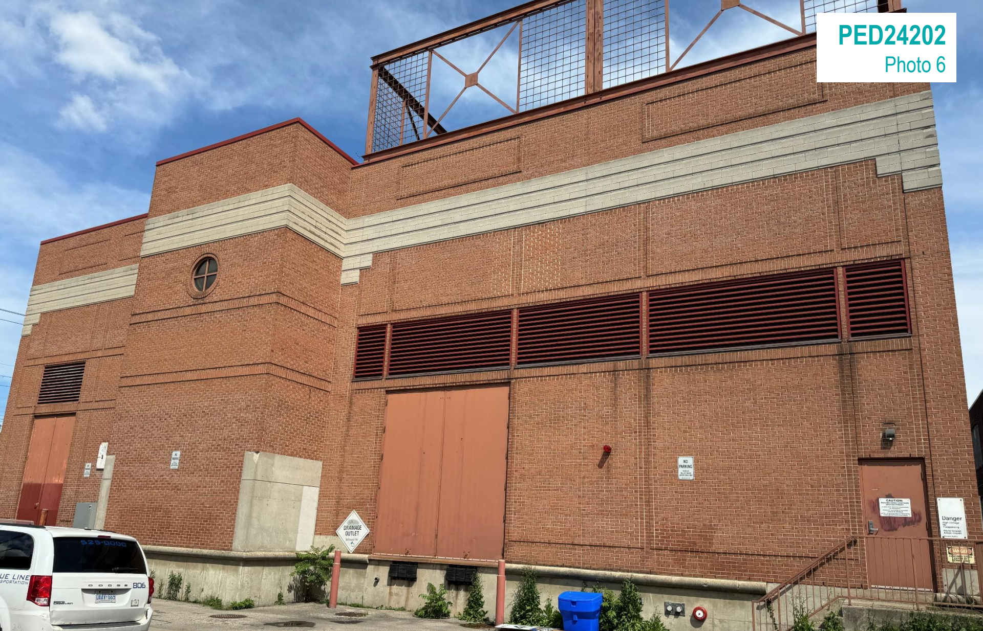
Property at 82 Stirton Street (Hydro Substation) located to the north of the Subject Lands, as seen from Stirton Street looking east
