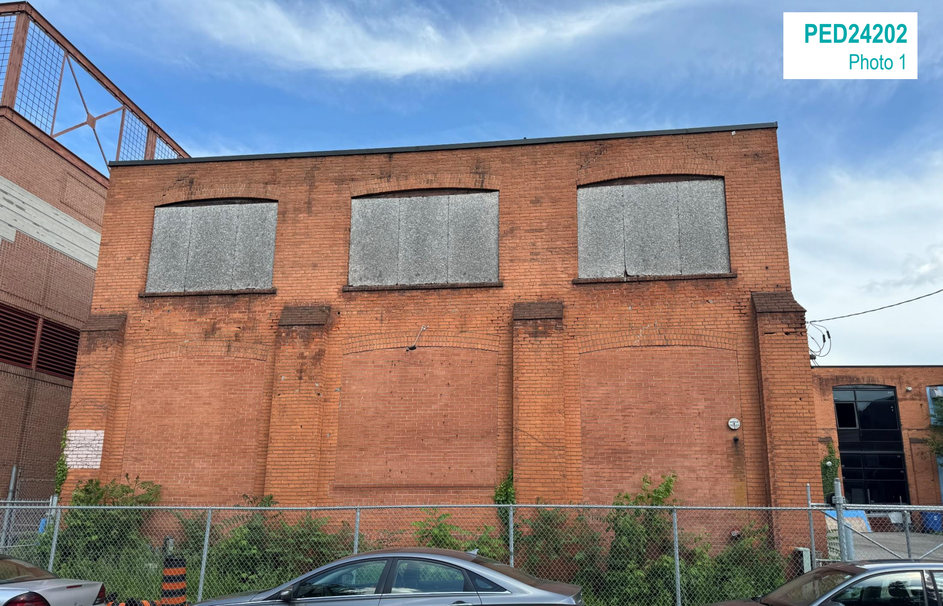
Subject Lands, as seen from Stirton Street looking east
