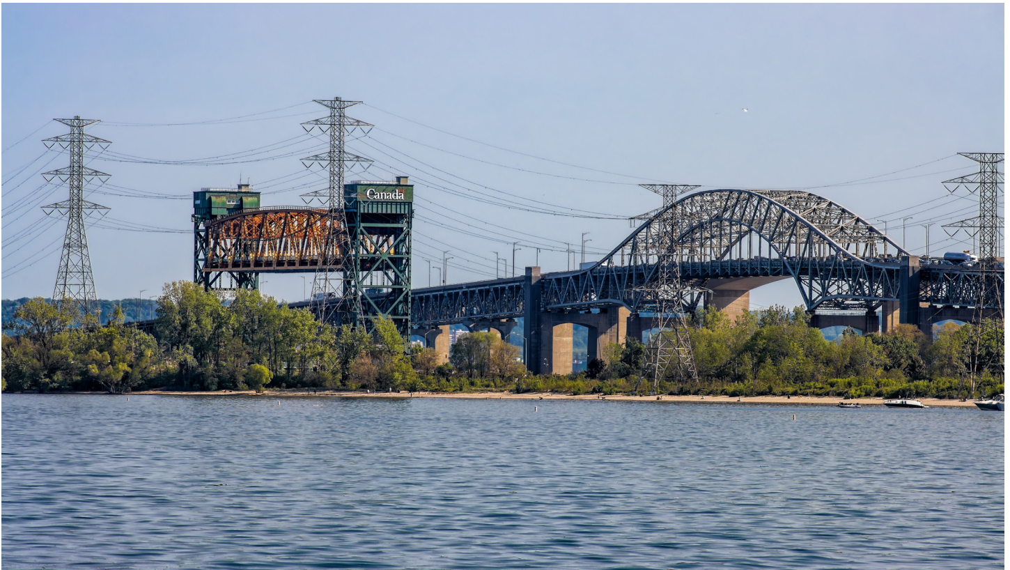
Burlington Canal Lift Bridge. STOCK PHOTO
