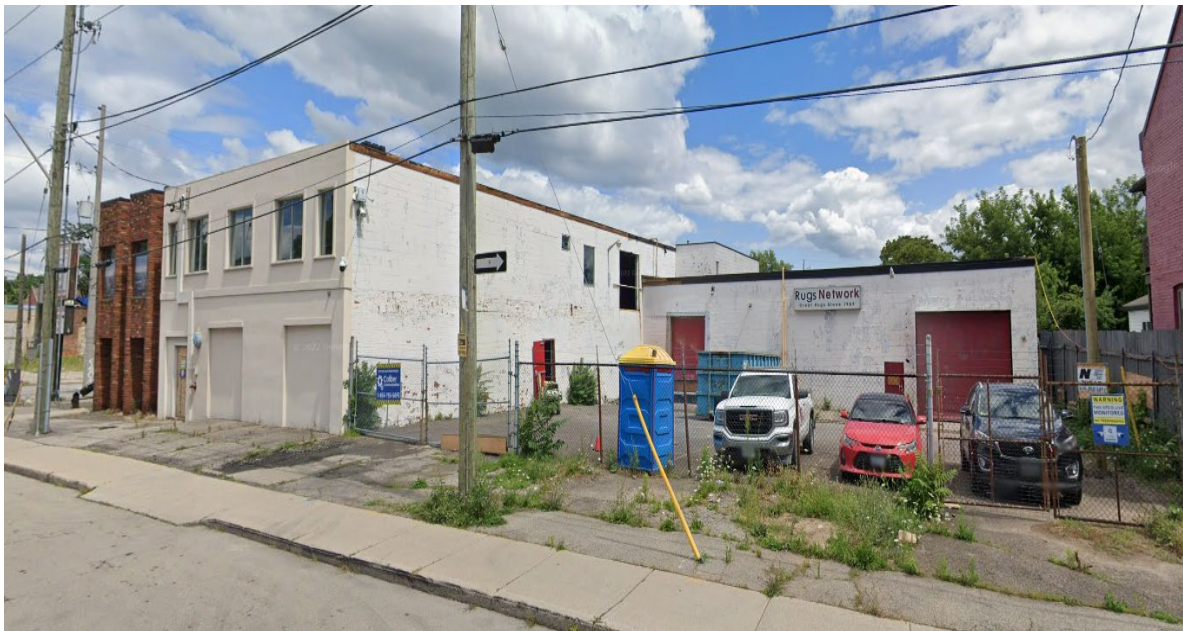
View looking north east toward the western elevation (Source: maps.google.ca; image from April 2022)
