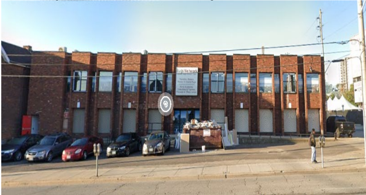
View looking south toward the northern elevation
