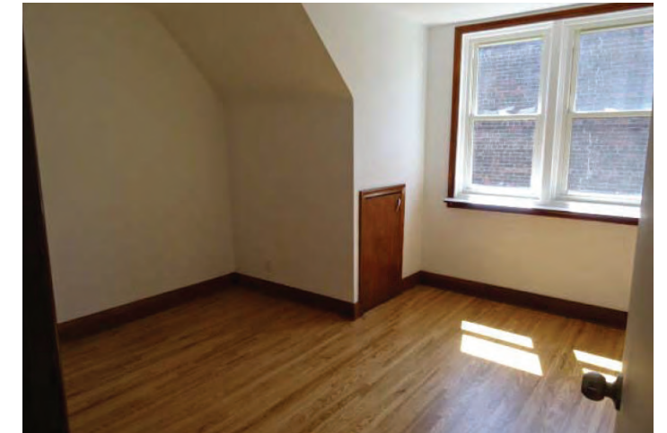
View of Level 3 under roof space with attic access door, wood trims and wood flooring. [Source: Aventus]
