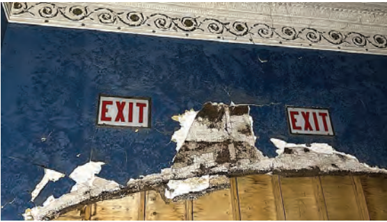
Photo 8: Example of exit signs suspected to contain lead acid batteries.
