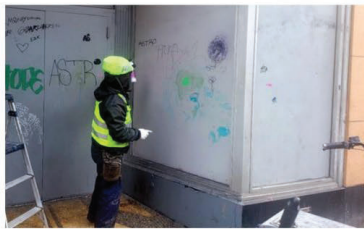
Clean Team Sidewalk / Graffiti Cleaning
