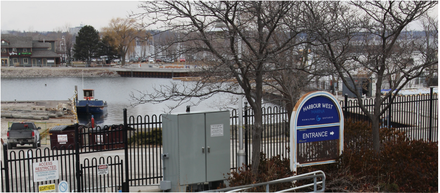
James Street North Combined Sewer Overflow Tank. PHOTO City of Hamilton.
