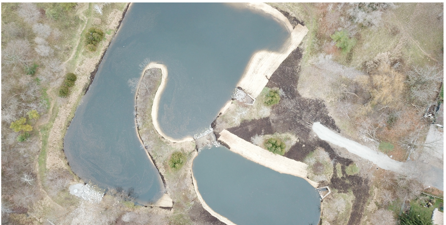
Delsey Stormwater Management Pond. PHOTO City of Hamilton
