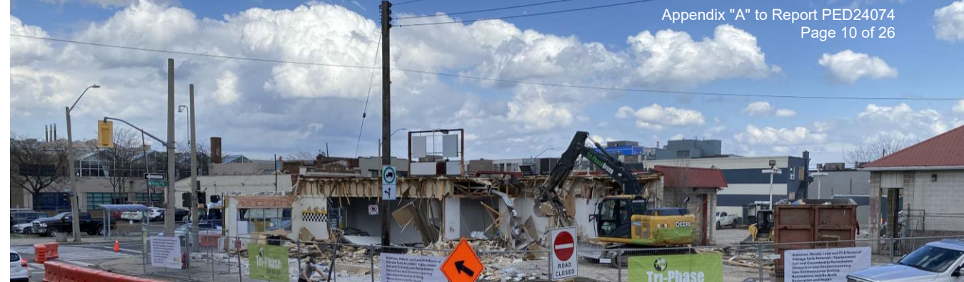
Demolition at King and Wentworth Streets
