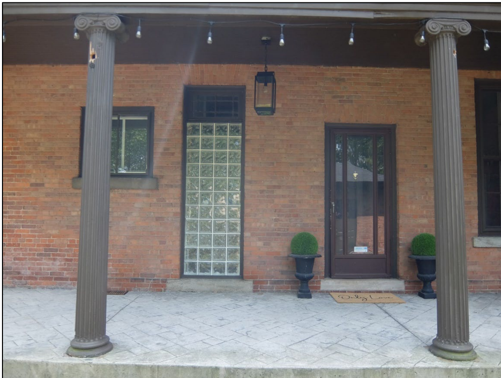
Figure 12: Closeup of northeast elevation entryway
