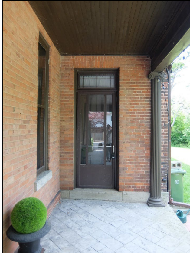
Figure 13: Northeast elevation entryway
