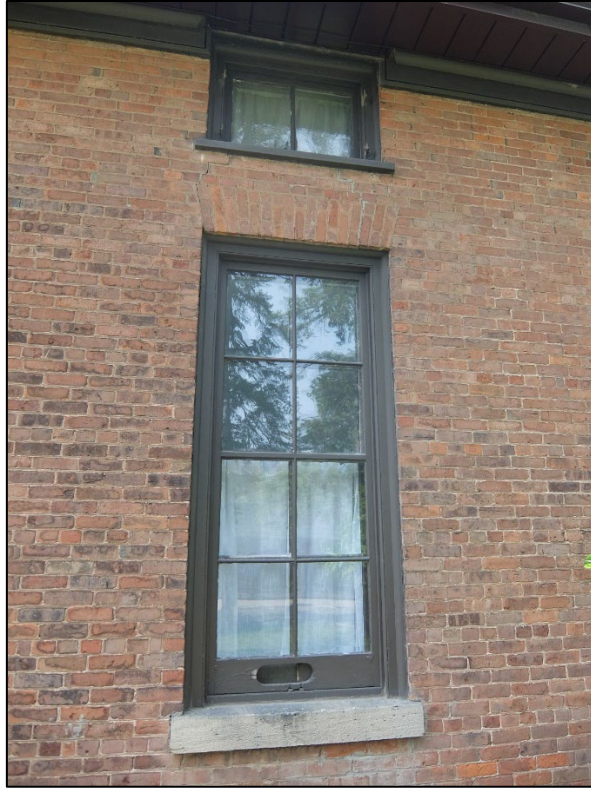
Figure 11: Closeup of east elevation windows
