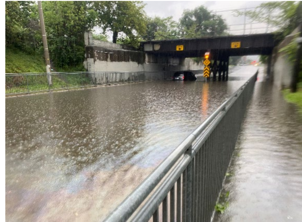
August 2023 – Birch Avenue flooding
