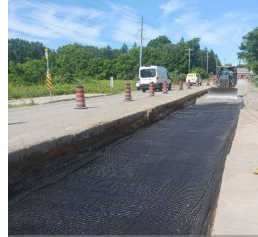
Garner Road: geo-grid installation
