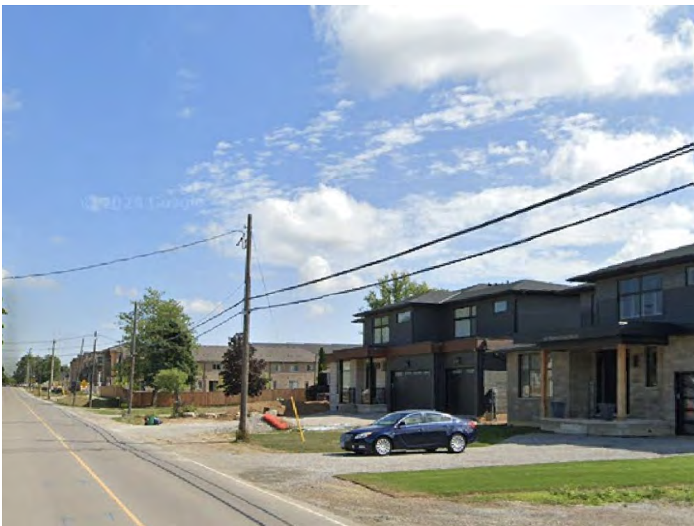
Figure 3: Street view north of subject properties (Google Streetview)
