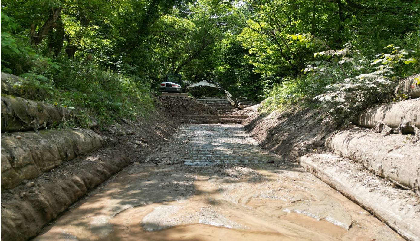
Sydenham Creek Retaining Wall:
