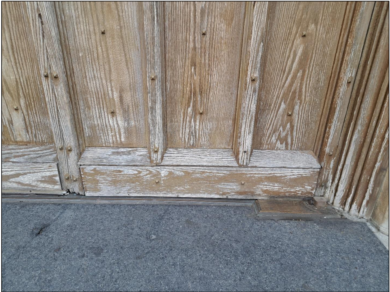
Figure 2: Heaving door jam and stile to be repaired
