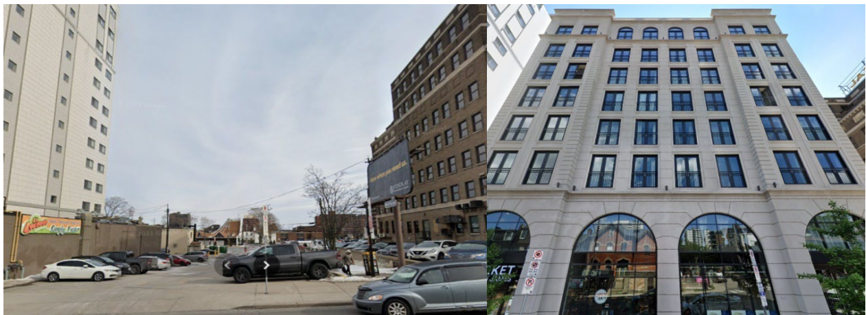
Previous and Post Development Condition – Building Two (February 2021/June 2024) – 165 Street South, Hamilton viewed looking east from James Street South (Source: maps.google.ca)
