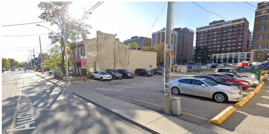
Previous Condition (October 2020) – 18 Augusta Street, Hamilton viewed southeast from Augusta Street (Source: maps.google.ca)
