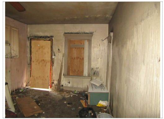
**PHOTO NUMBER: 7** Typical conditions of second floor **Note:** Abandoned belongings, moisture stains on walls
