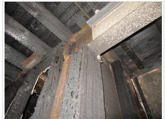
**PHOTO NUMBER: 5** Interior of main floor of building (underside of second floor). **Note:** Area of burnt floor joists, burnt framing walls.
