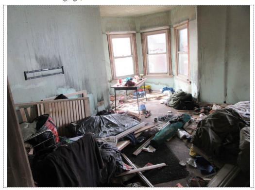
**PHOTO NUMBER: 8** Typical conditions of second floor **Note:** Abandoned belongings, moisture stains on walls
