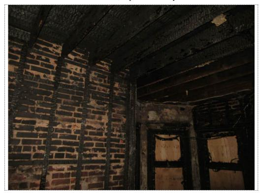
**PHOTO NUMBER: 4** Interior of main floor of building (underside of second floor). **Note:** Area of absent/burnt interior walls, exposed masonry, burnt floor joists.
