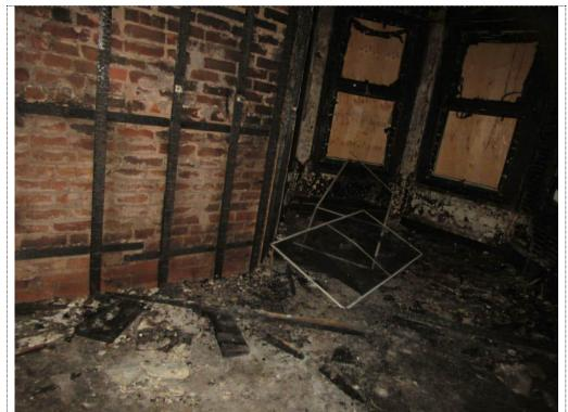
**PHOTO NUMBER: 3** Interior of main floor of building **Note:** Area of absent/burnt interior walls, exposed masonry.
