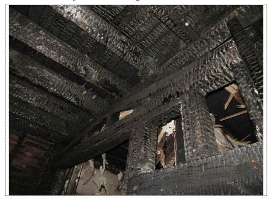
**PHOTO NUMBER: 6** Interior of main floor of building (underside of second floor). **Note:** Area of burnt floor joists, burnt framing walls.
