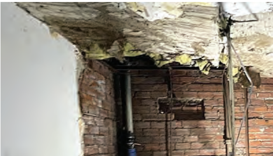
Photo 11: Water damage and mould growth in staircase area leading to projection room.
