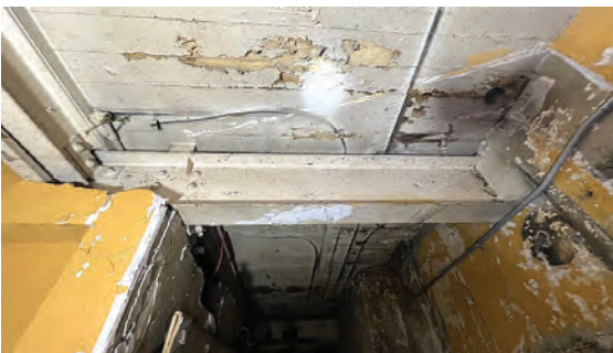
Photo 1: Example of peeling and flaking paint on wood ceilings below stage area.
