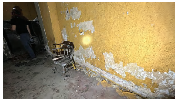
Photo 2: Example of peeling and flaking paint on plaster walls below stage area.
