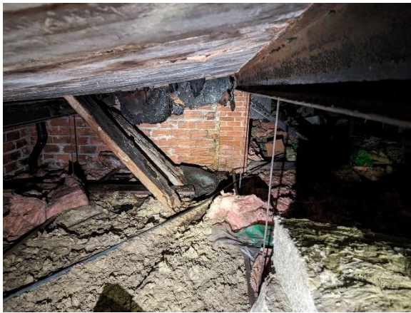
Fig 3: Pier separation, from attic, in Jan 2024.
