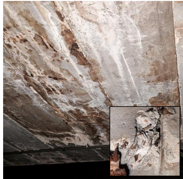
Fig. 6: Roof deck, inset w/ panel composition
