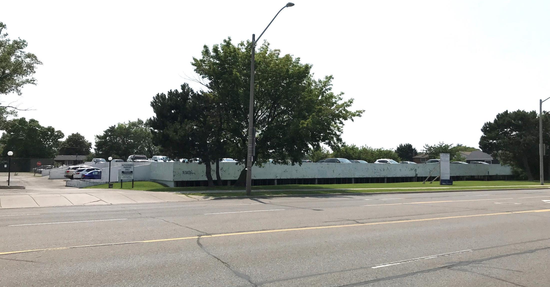
Subject site – existing parking structure
