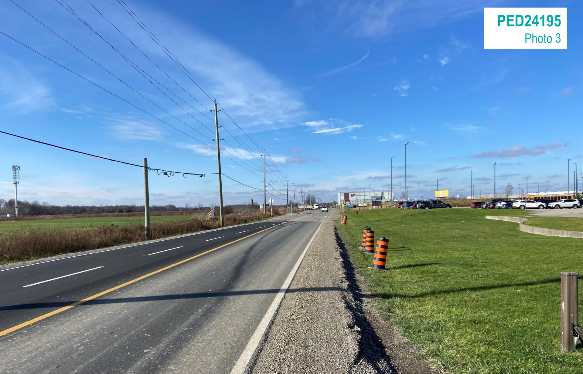
Airport Road West looking west
