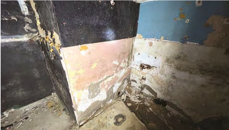
Example of moisture damage on lower walls throughout rooms below stage area.
