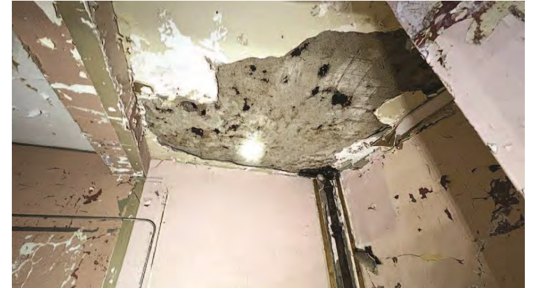
Water-damaged ceiling and mould growth on second floor.
