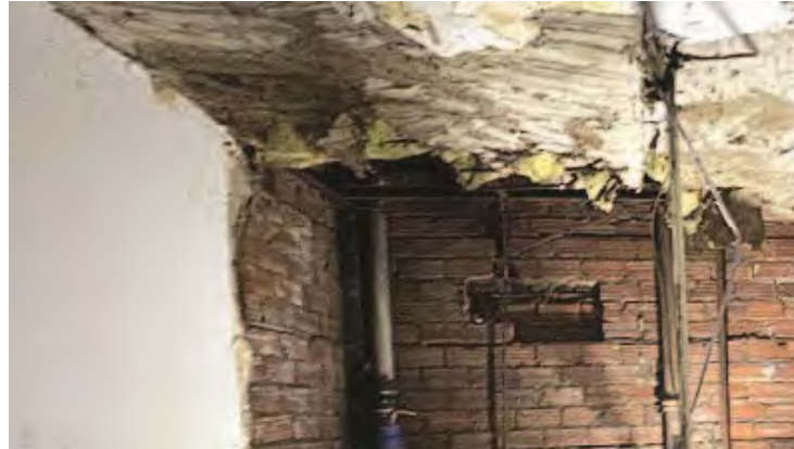
Water damage and mould growth in west corner of south elevation, seen from the second floor.
