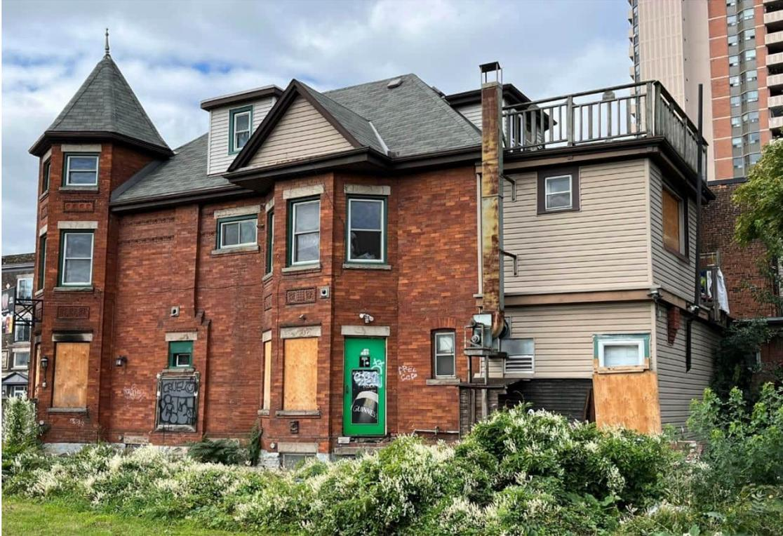
**Photograph 7: Chimney window with terra cotta projecting header and apron (AECOM, October 2024)**
