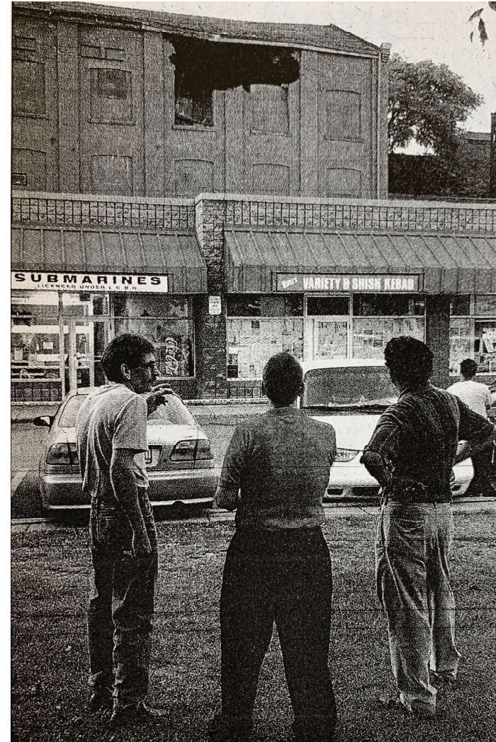
Passerby observe the damage in the Tivoli wall [Source: Hamilton Public Library]
