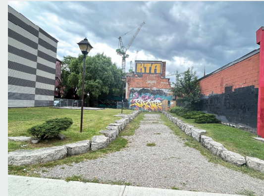
Tivoli Theatre site - View from James St N looking at the remaining entrance. [Source: +VG Architects]
