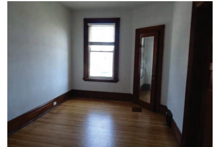
View of Level 2 bedroom with historic wood trim, baseboards and wood flooring. [Source: Aventus]
