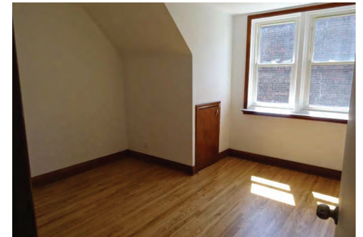
View of Level 3 under roof space with attic access door, wood trims and wood flooring. [Source: Aventus]
