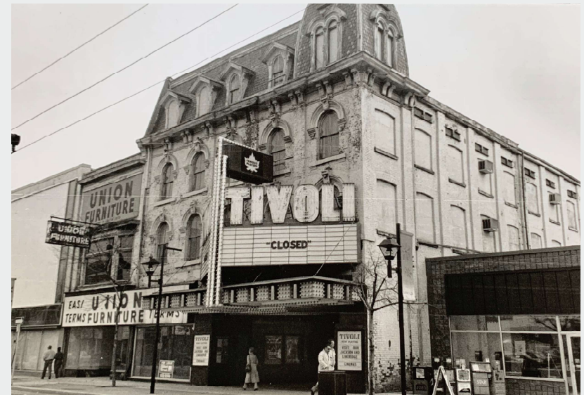
Tivoli Theatre - Front Facade [Source: Hamilton Public Library]
