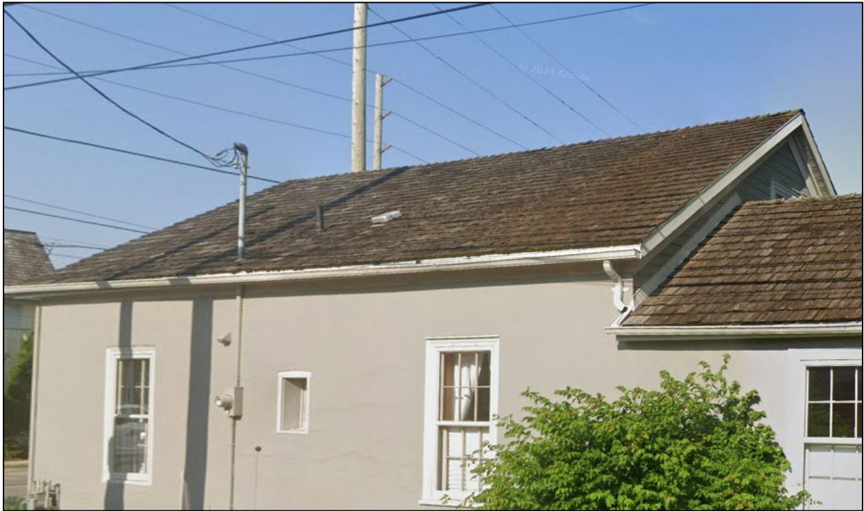
Figure 4: West elevation, showing front portion of home and roof
