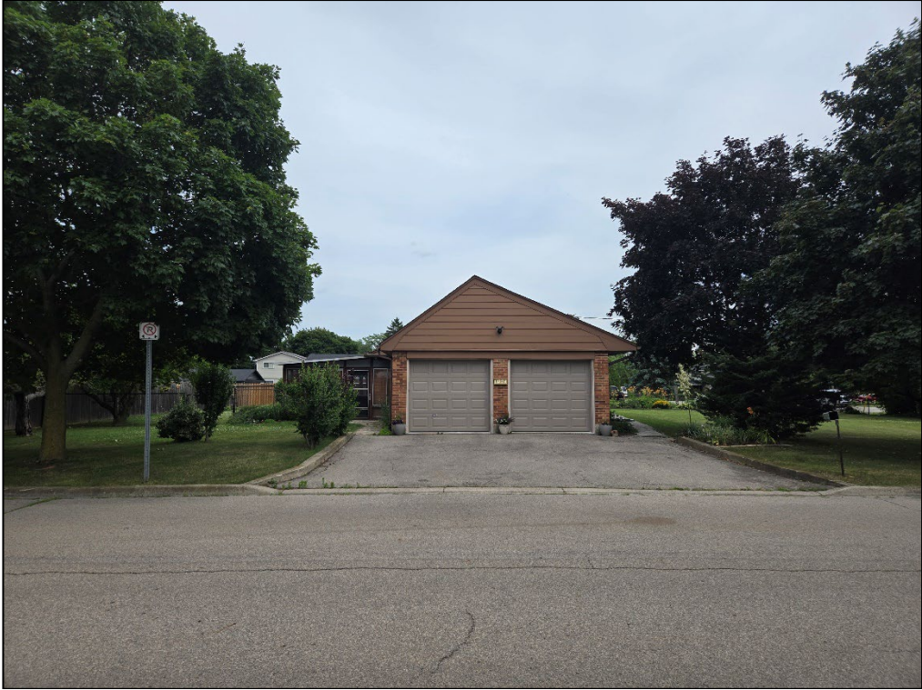
Figure 5 - 1341 Highway 8 – Across from the Subject Lands (East)
