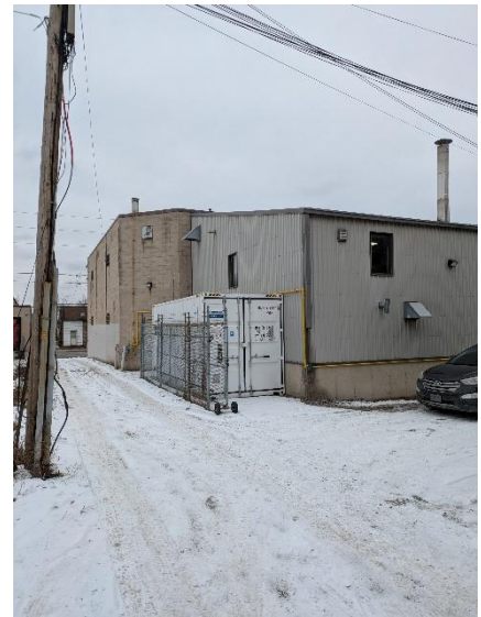
Electric Motor Service (EMS) from laneway
