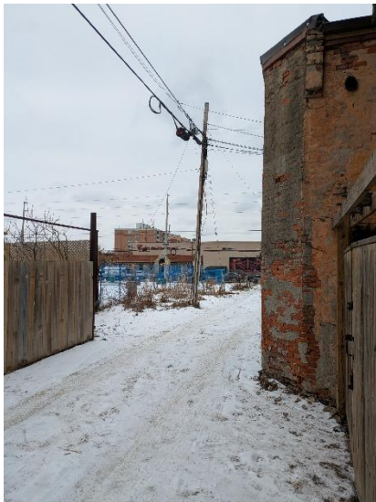
Laneway at 71 Cathcart looking towards site corner and utility pole
