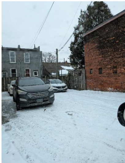
EMS Parking area and Coach House wall at 71 Cathcart
