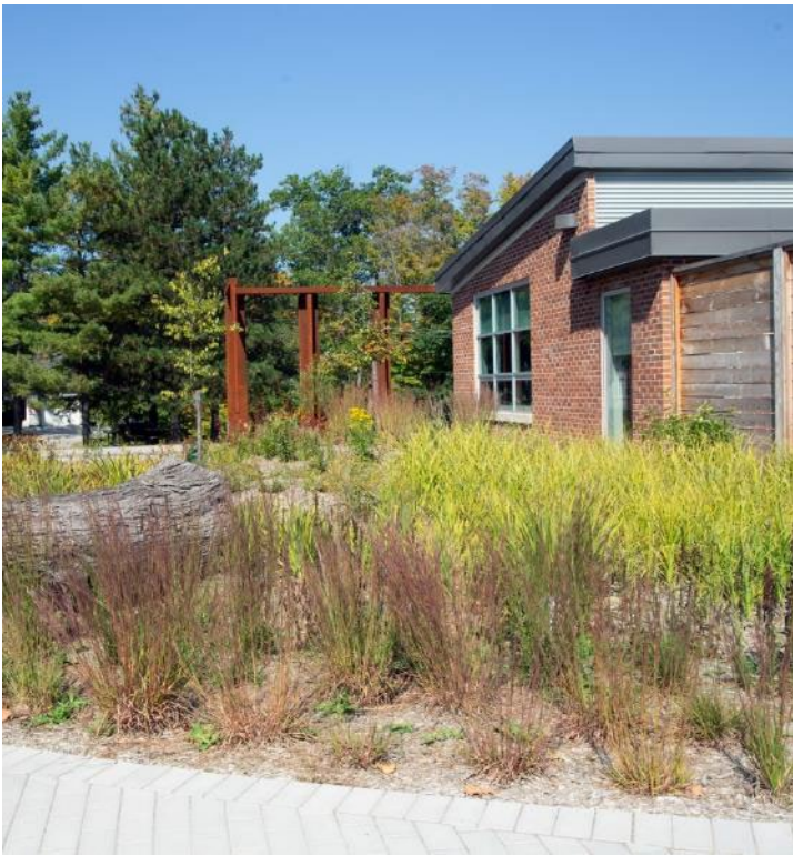
Low-impact development at Conservation Halton Administration
