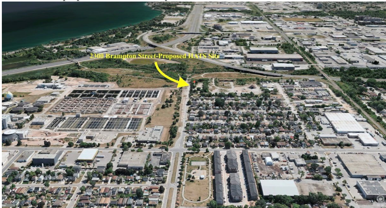
Aerial view of proposed site-2300 Brampton Street
