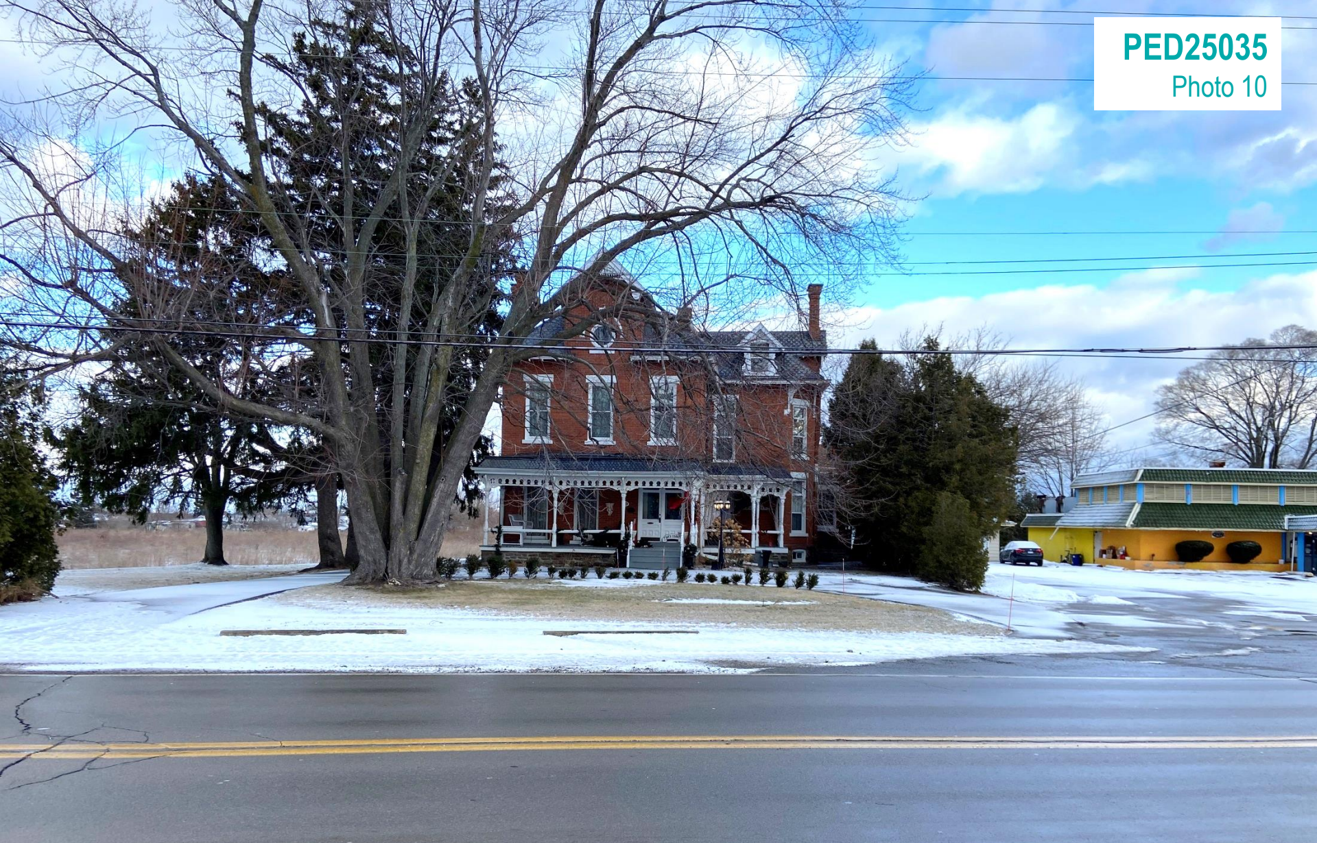
1059 Highway No. 8 (Carpenter House)
