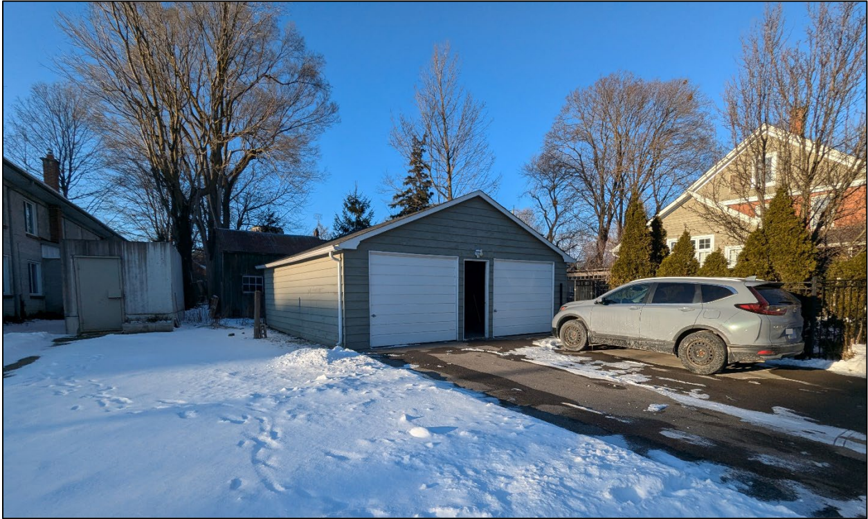
Figure 3: View of the Existing Garage and shed behind as seen from John Street (c.o. Site Visit, January 14, 2025)
