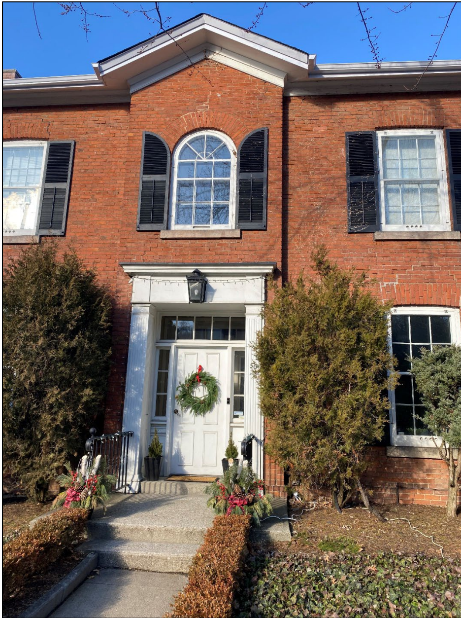
Figure 2: View of the Property from Markland Street (c.o. Site Visit, February 13, 2023)
