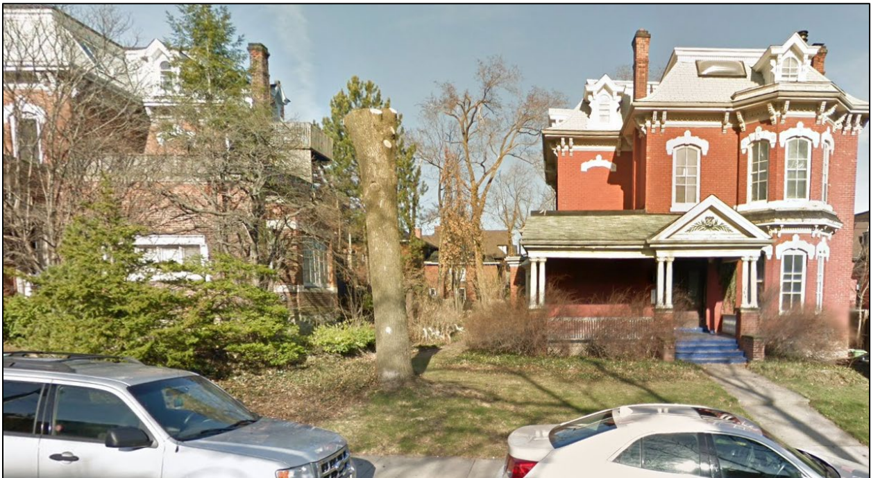
Figure 4: View of the existing rear addition from MacNab Street (Google Street View)
