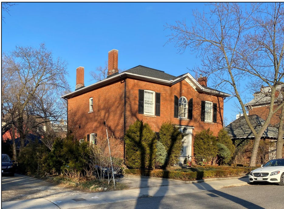
Figure 2: View of the Property from Markland Street (c.o. Site Visit, February 13, 2023)
