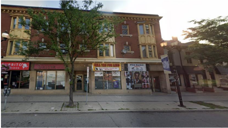
Figure 5 – Street View of Mixed-Use Buildings to North of Subject Property
