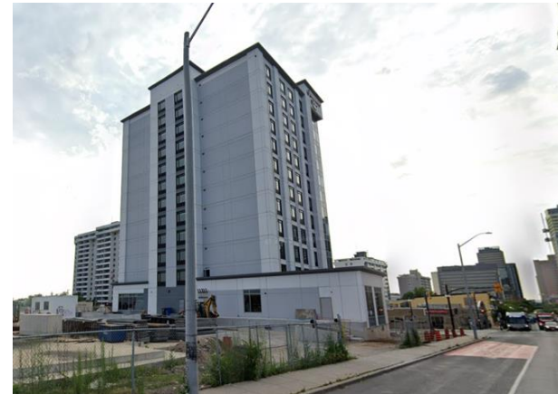
Figure 10 – Hampton Inn (NW Corner of King Street/Queen Street North)
