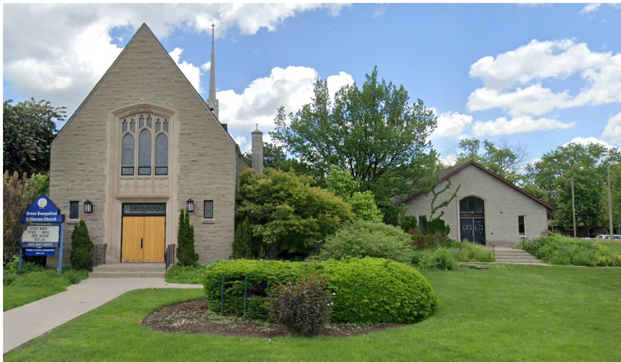
Figure 2: Existing Church Building (Source: Google Earth)
