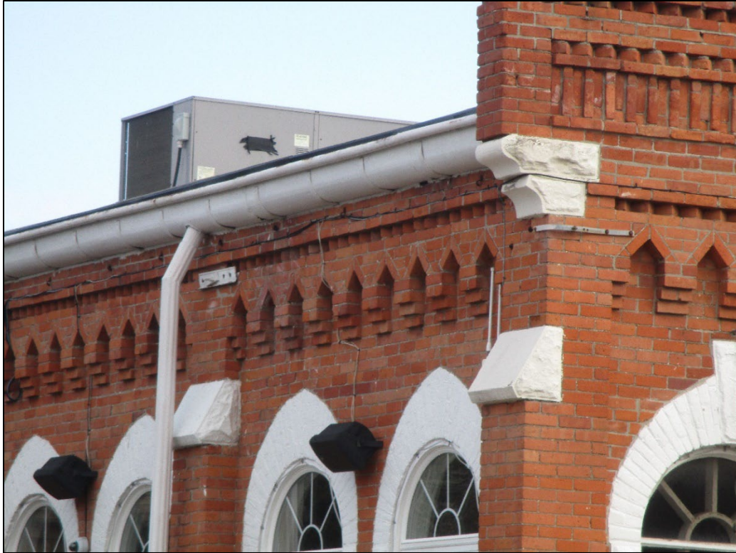
Figure 11: Detail view of butress capstones and stone corbel on southwest corner.
