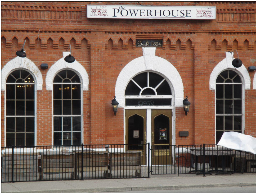
Figure 6: Detail view of windows and doorway on south elevation.
