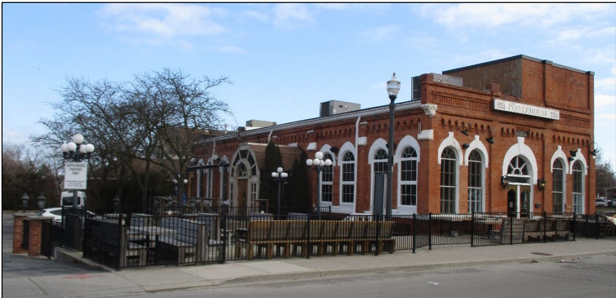
Figure 2: South and west elevations of subject property.
