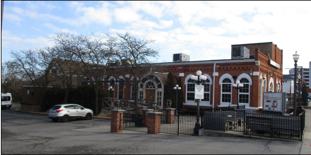
Figure 3: West elevation showing modern entrance.
