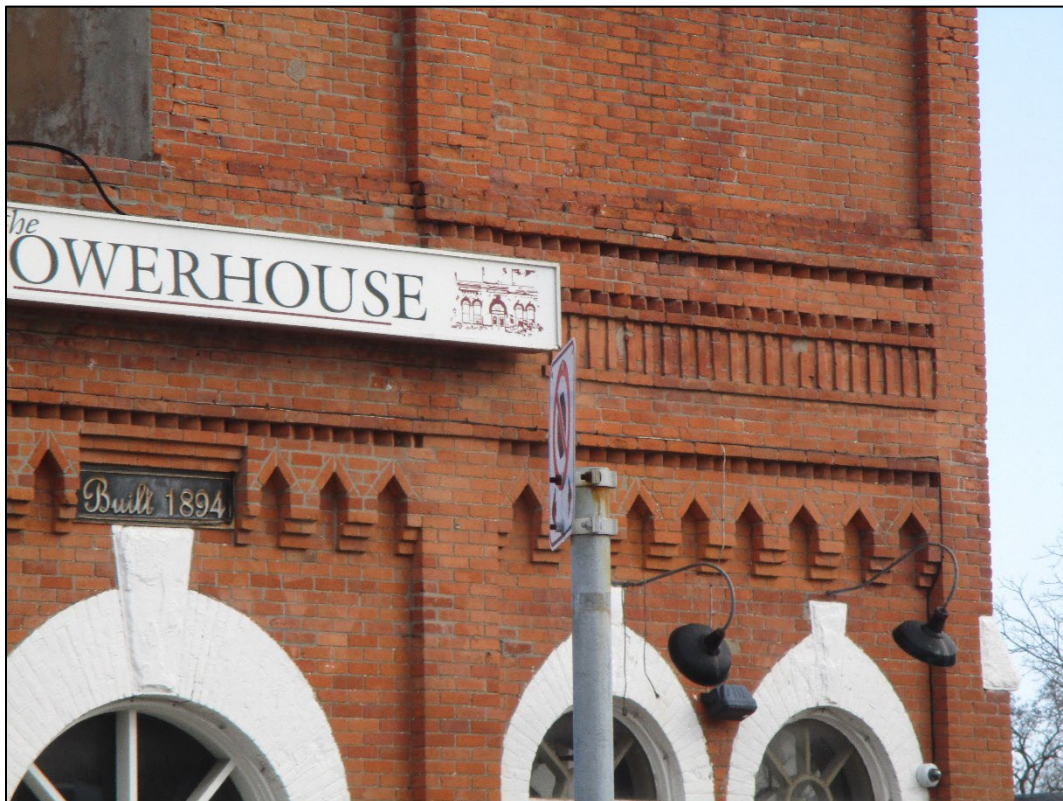
Figure 8: Detail view of decorative brickwork elements.
