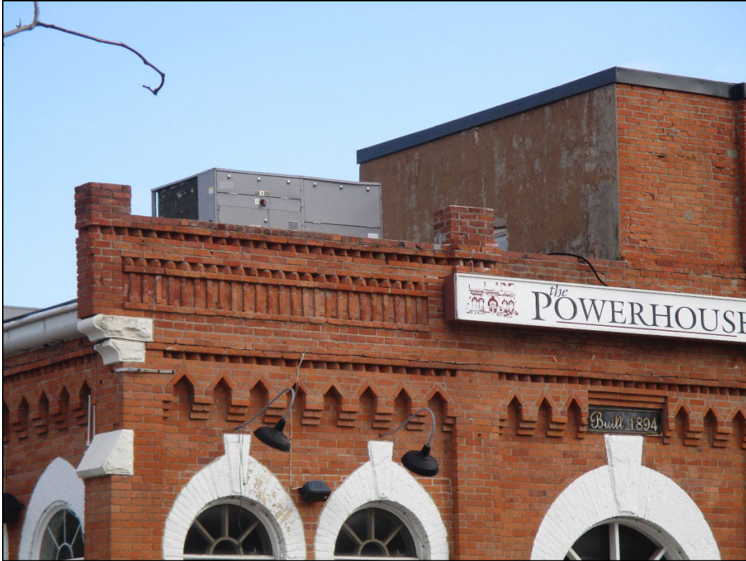
Figure 7: Detail view of parapet with decorative brickwork.
