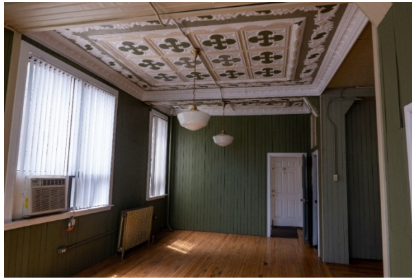
Figure 12: View of wood strip paneling on walls and tin ceilings in the office.
