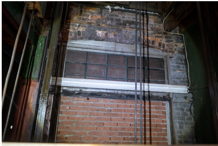
Figure 50: Former transom window remains visible inside Section B.
