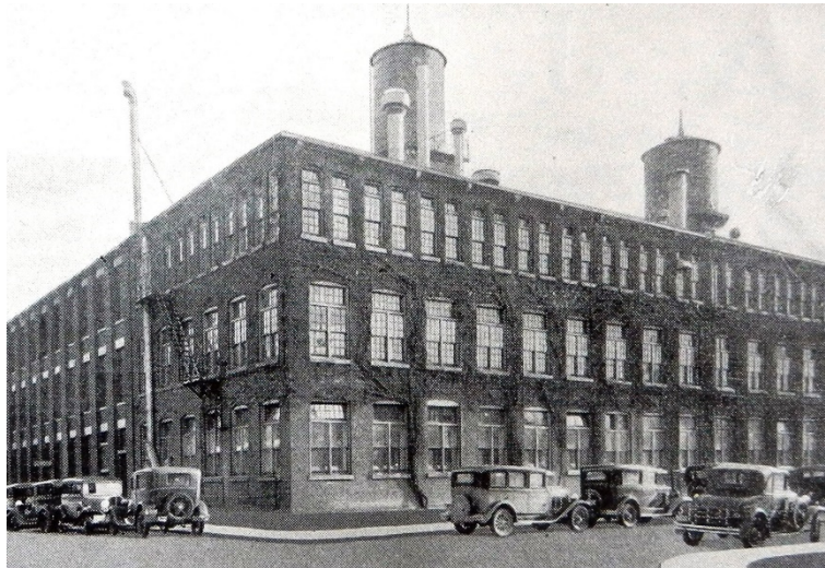
Figure 44: Photograph of the c.1911 American Can Company Factory, Hamilton, ON, showing the use of repeating bays as organizing principle ( https://mackerel-semicircle-g65b.squarespace.com/american-can-company ).
