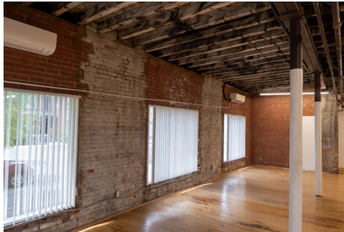
Figure 37: View of Section Z addition interior space, with steel beam and different ceiling structure.
