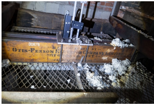
Figure 19: Otis-Fensom top beam of the elevator car.
