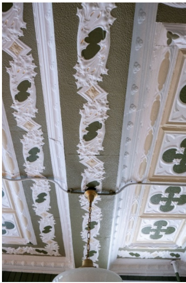
Figure 13: Detail of tin panel ceiling.
