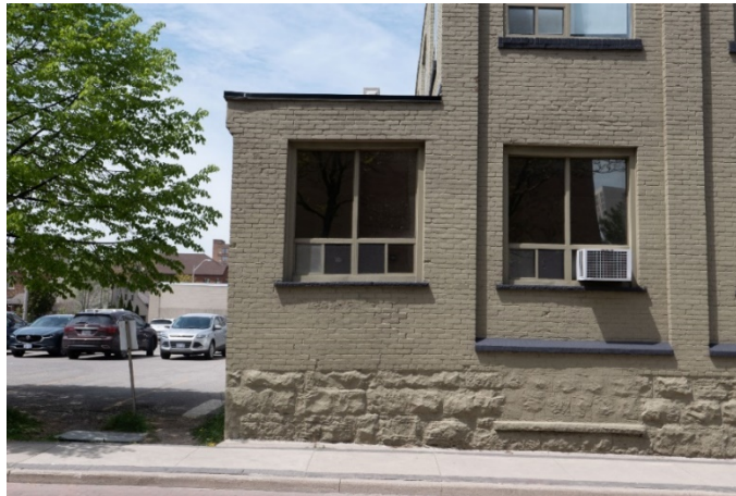
Figure 6: Non-original flat window openings seen on south end of the main elevation and south addition.
