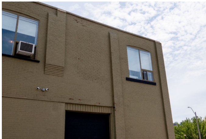
Figure 7: Infilled former window openings at the south end of the west elevation, on both stories.
