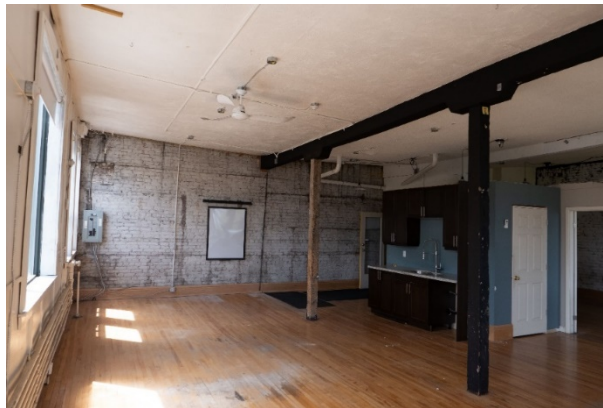
Figure 20: View of party wall and wooden posts at the second floor level.
