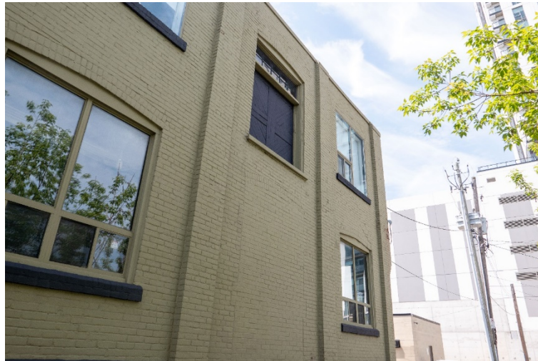
Figure 49: Former openings taller than windows at grade, and the remnant door above suggest loading functions related to the elevator .
