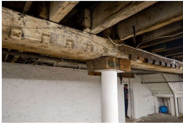
Figure 23: Salvaged wood beams and round posts under the original portion of 48 Ferguson.
