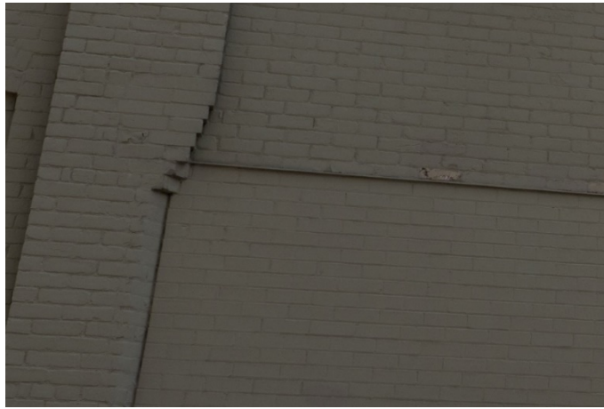
Figure 35: Brick details of Section B (left) partially obscured by the subsequent Section C addition.
