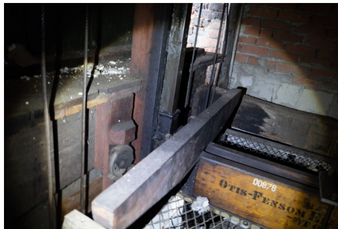
Figure 53: View of the elevator's wooden guide posts.
