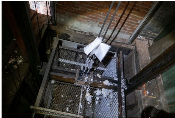
Figure 52: View of the elevator's open freight car.
