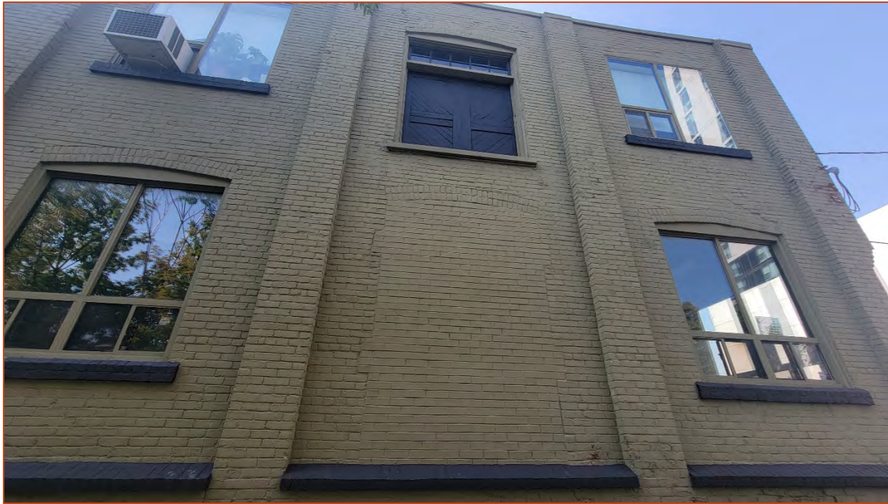
Photo 9. View of the second-storey freight elevator opening and the infilled opening on the first storey of the north elevation of the Radigan Building.
