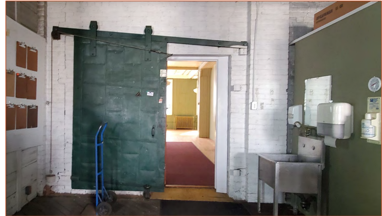
Photo 23. View of the metal sliding fire door and entrance to the rear workshop area.
