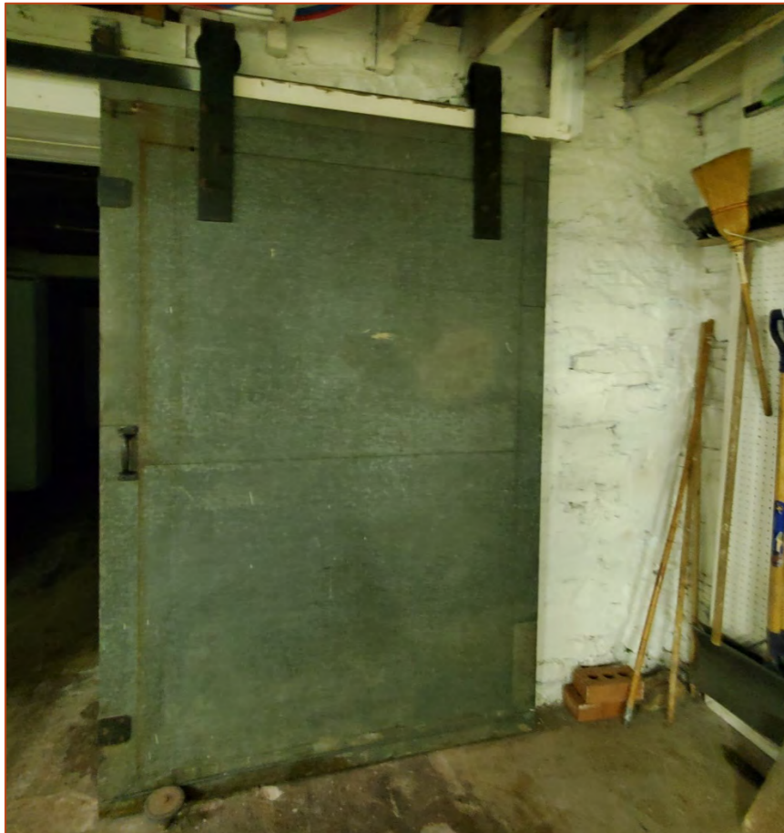
Photo 14. View of a metal sliding fire door in the basement.
