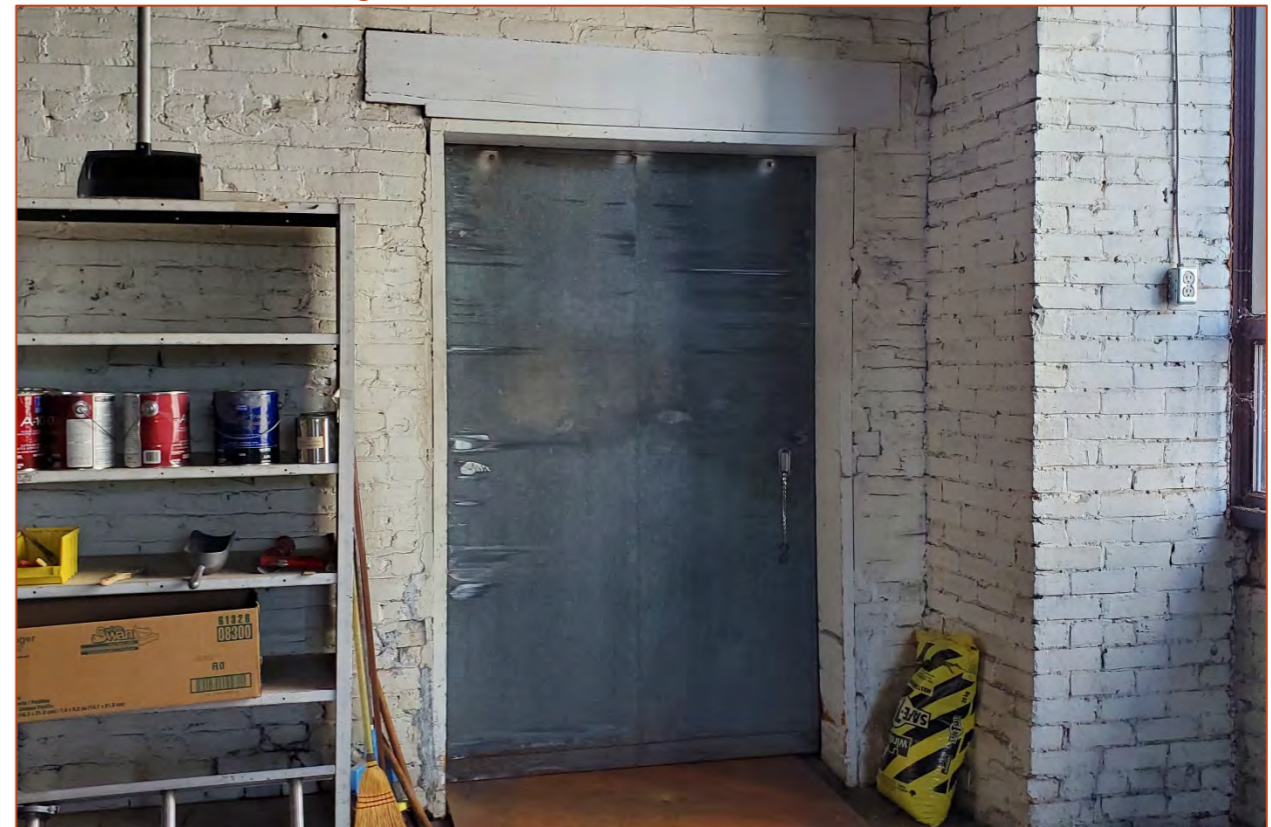
Photo 32. View of a metal door and a wood lintel.
