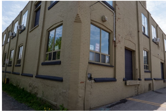
Figure 8: Decorative corbelling transitioning chamfered northwest corner.
