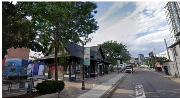
Figure 61: View of the interpretive train station gazebo building in Ferguson Station Park (Google 2022).
