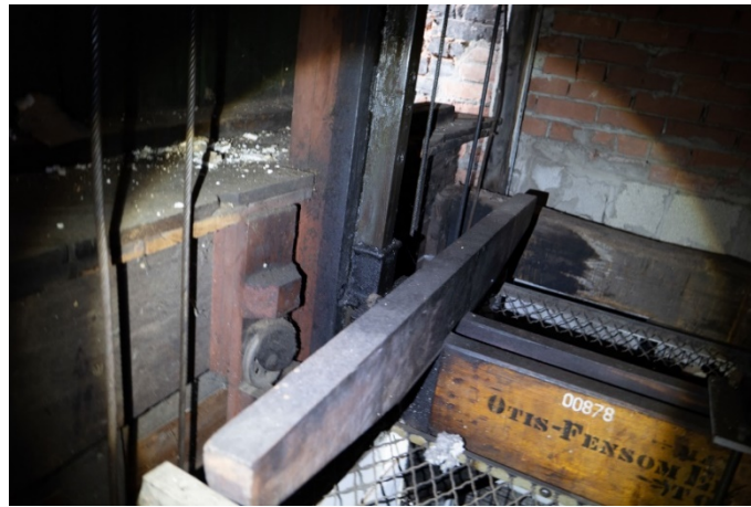
Figure 53: View of the elevator's wooden guide posts.
