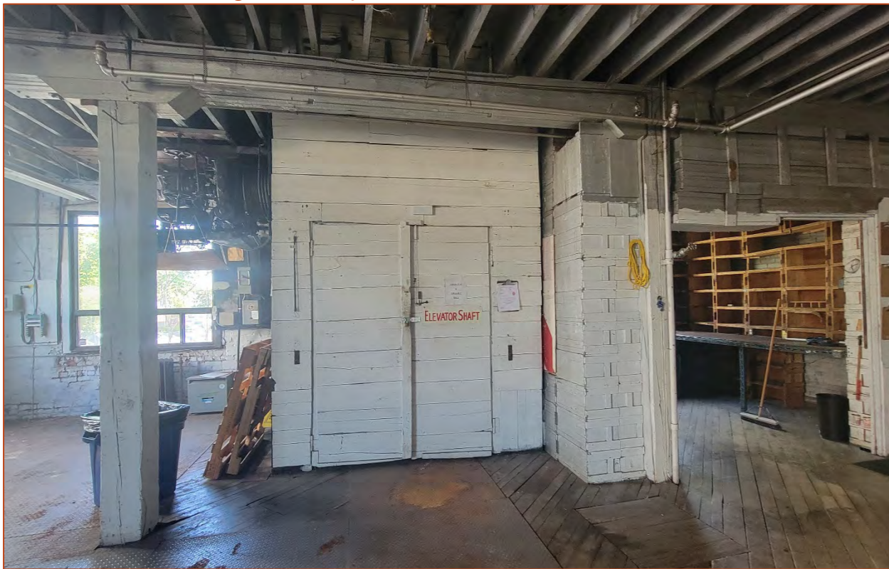
Photo 26. View of the closed 1909 wooden freight elevator shaft.
