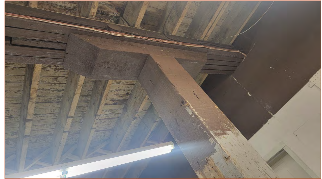
Photo 35. Enlarged view of a timber post and timber beam.
