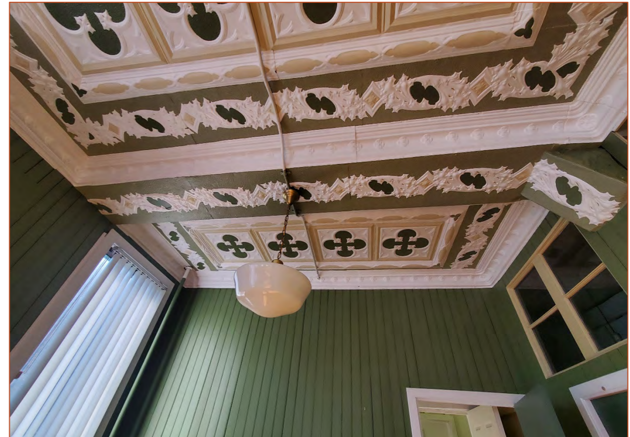
Photo 20. View of the decorative relief aluminium ceiling.
