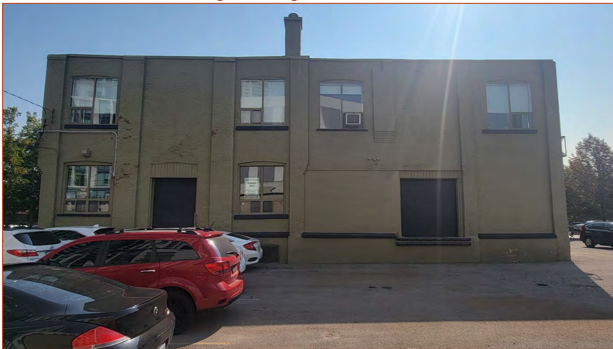
Photo 10. View east of the west elevation of the Radigan Building.
