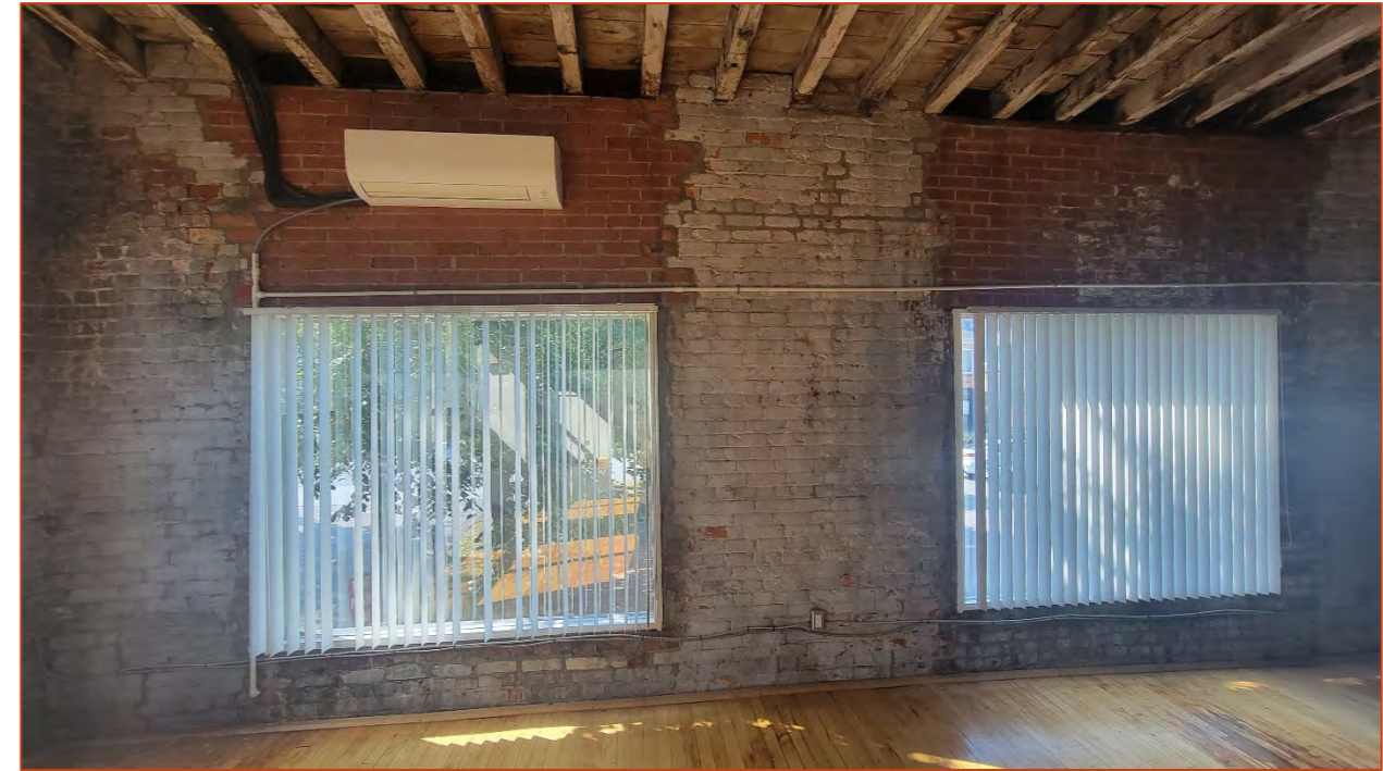
Photo 39. View of two windows and exposed brick wall.
