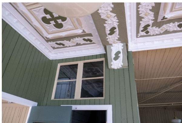
Figure 14: Office details, including transom window and tin panel ceiling.
