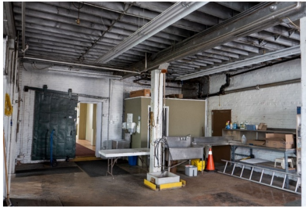
Figure 15: Rear workshop space of 46 Ferguson, with former filled in window openings visible at rear.
