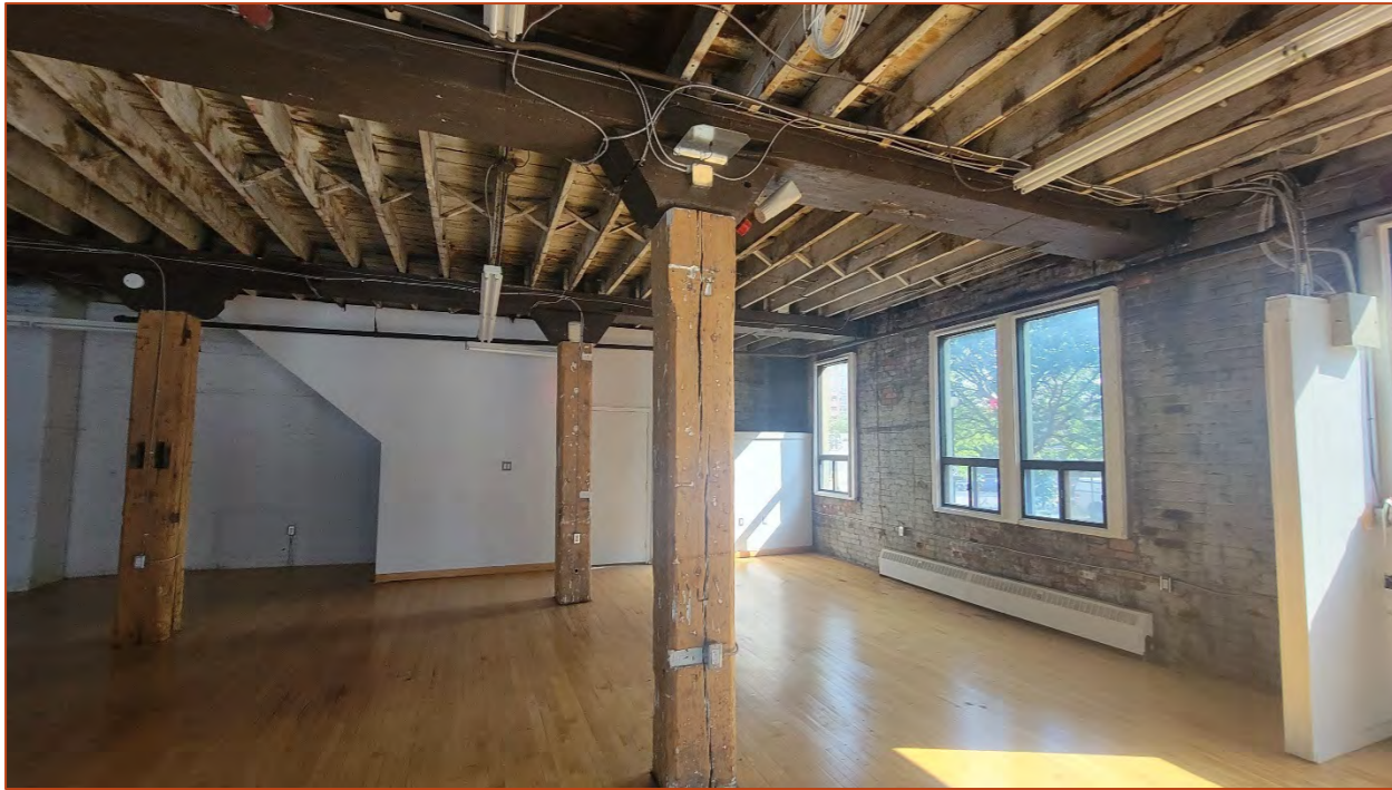
Photo 37. View of a large room with timber posts and timber beams.
