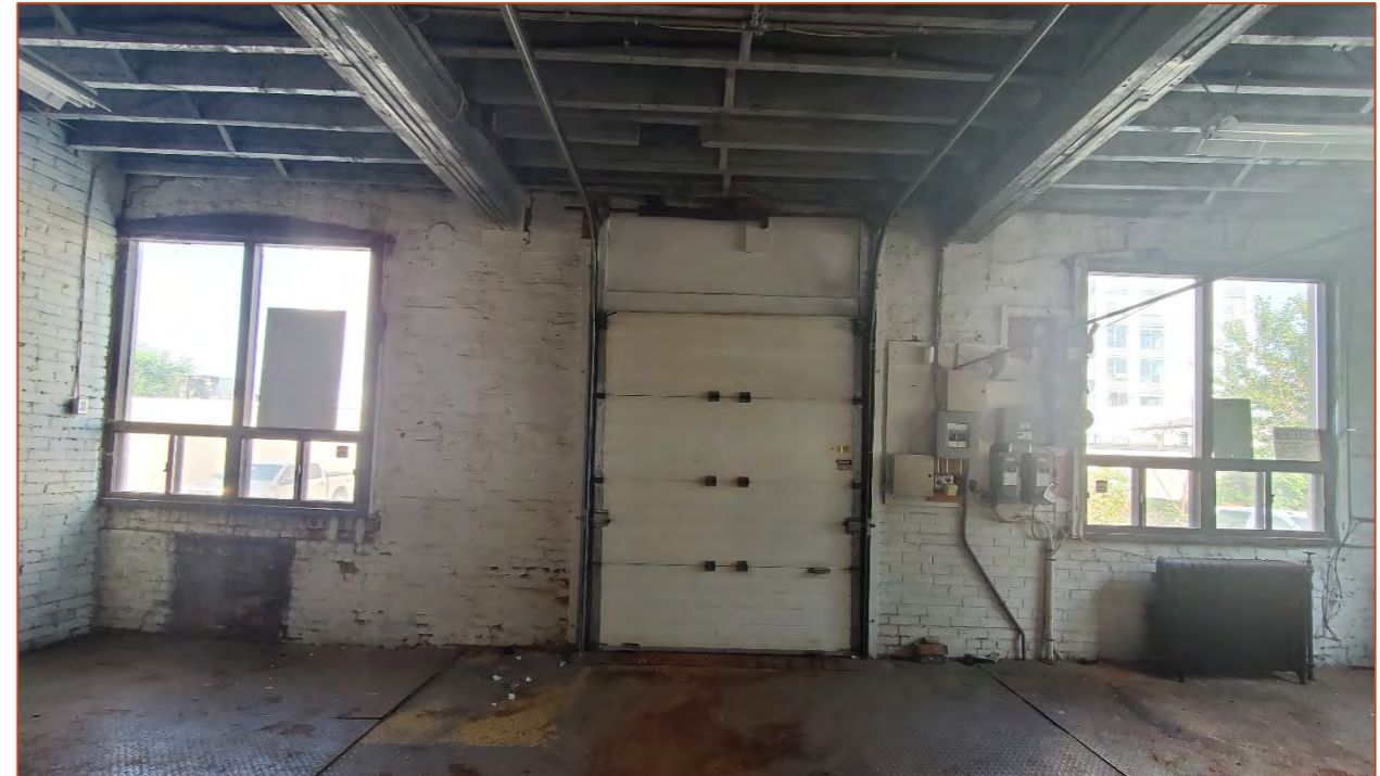
Photo 31. View of a loading door at the rear.
