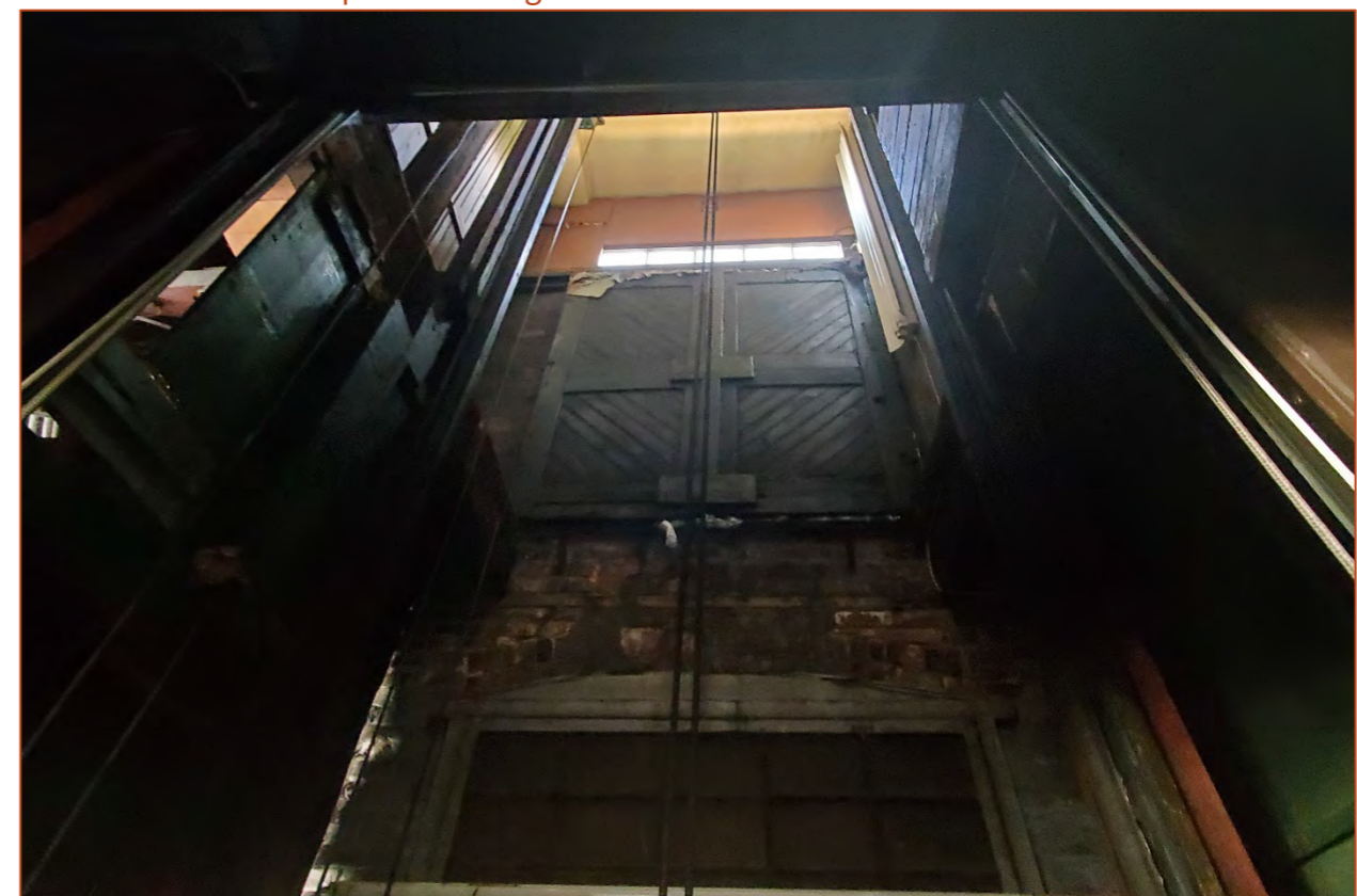
Photo 28. View of the 1909 freight elevator shaft looking towards the second floor.
