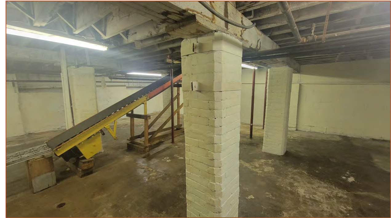
Photo 15. View of a partitioned room with a conveyor belt and wooden beams supported by chamfered brick pillars.
