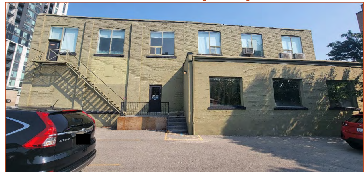
Photo 12. View north of the south elevation of the Radigan Building.
