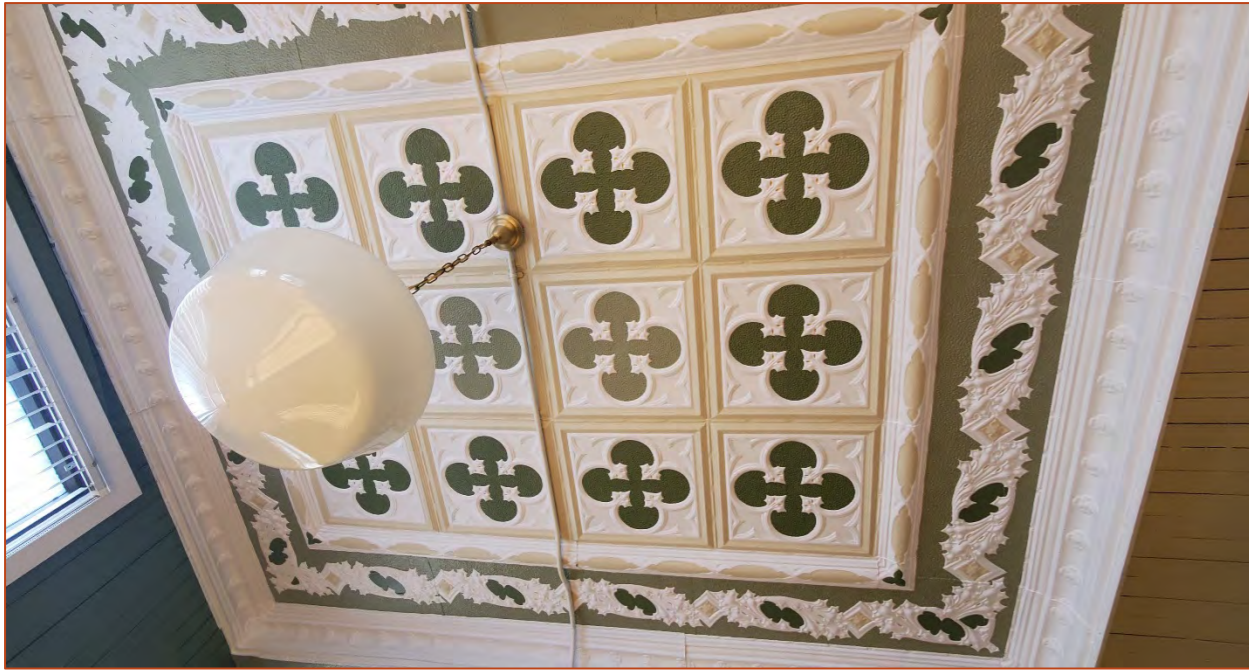
Photo 21. View of the decorative relief aluminium ceiling.
