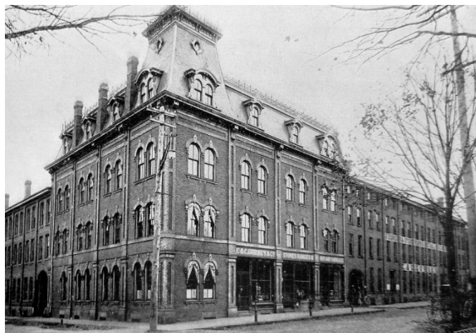
Figure 46: The E. & C. Gurney and Co. foundry, Toronto (demolished) added an elaborate Second Empire style office and showroom to their facilities in 1875 ( https://www.workerscity.ca/e-c-gurney-foundry ).
