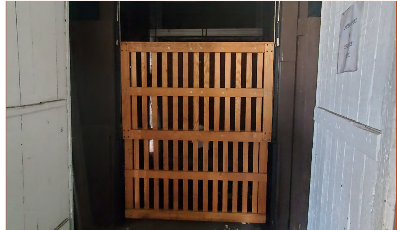
Photo 27. View of the open 1909 freight elevator shaft and elevator door.
