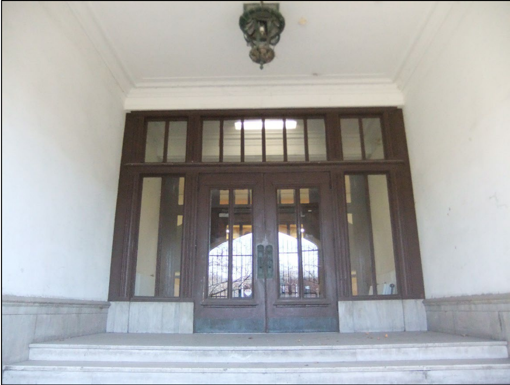
Figure 21: Detail view of doorway within main entrance.
