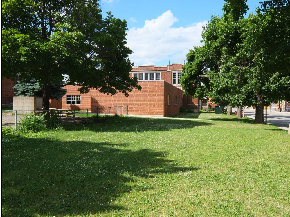
Figure 7: East side yard looking north, showing 1921 Manual Arts building and modern connecting annex. City of Hamilton staff, July 9, 2014.
