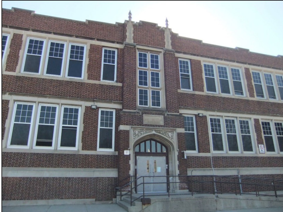
Figure 27: View of side entrance on west elevation.
