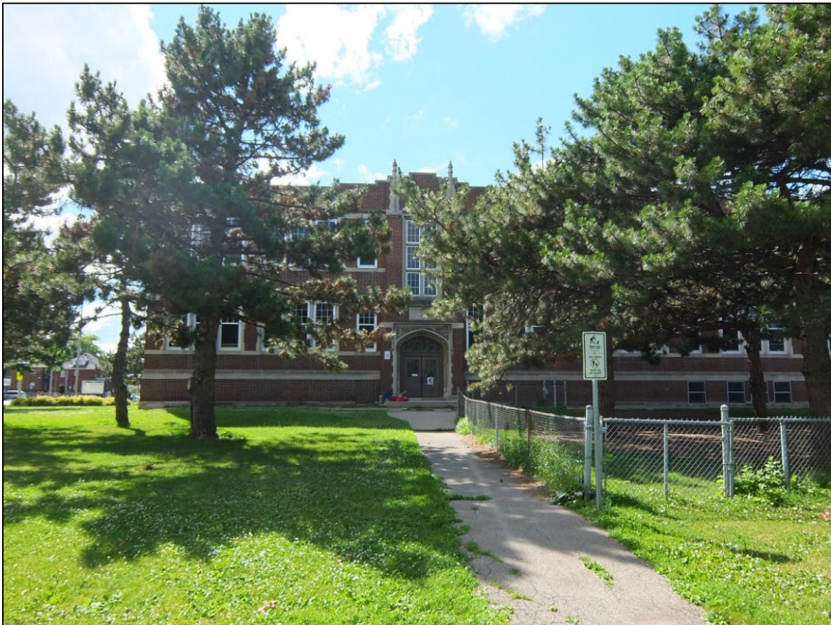
Figure 6: East side elevation, southern end. City of Hamilton staff July 9, 2014.
