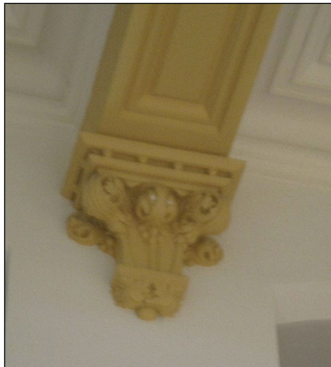
Figure 37: Detail view of bracket supporting coffered ceiling.
