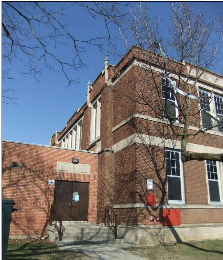
Figure 10: View of modern annex attached to 1921 Manual Arts building.
