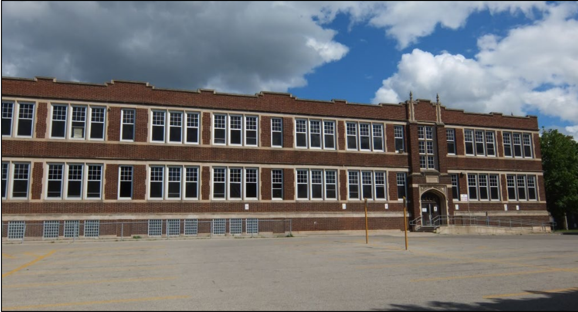
Figure 5: Western side elevation, southern end. City of Hamilton staff, July 9, 2014.
