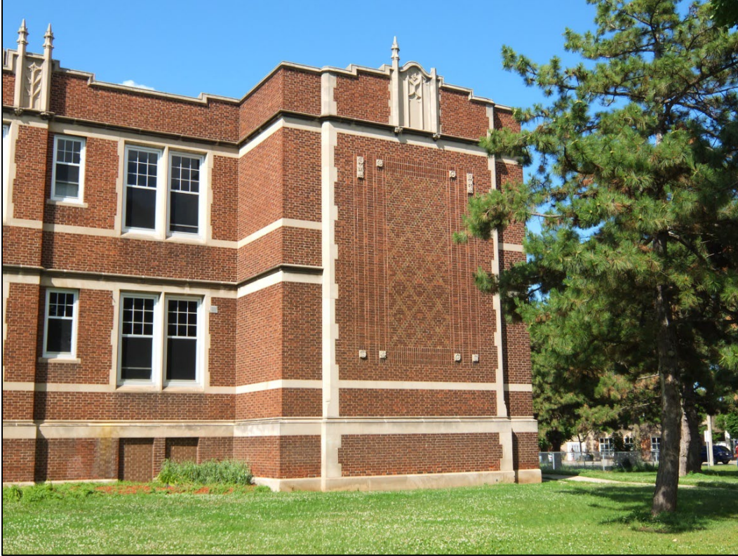
Figure 23: Decorative brick panels on south elevation. City of Hamilton staff, July 9, 2014.
