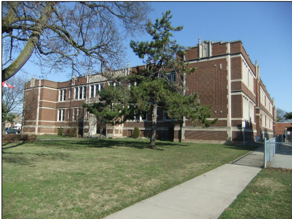
Figure 2: South elevation looking northwest.
