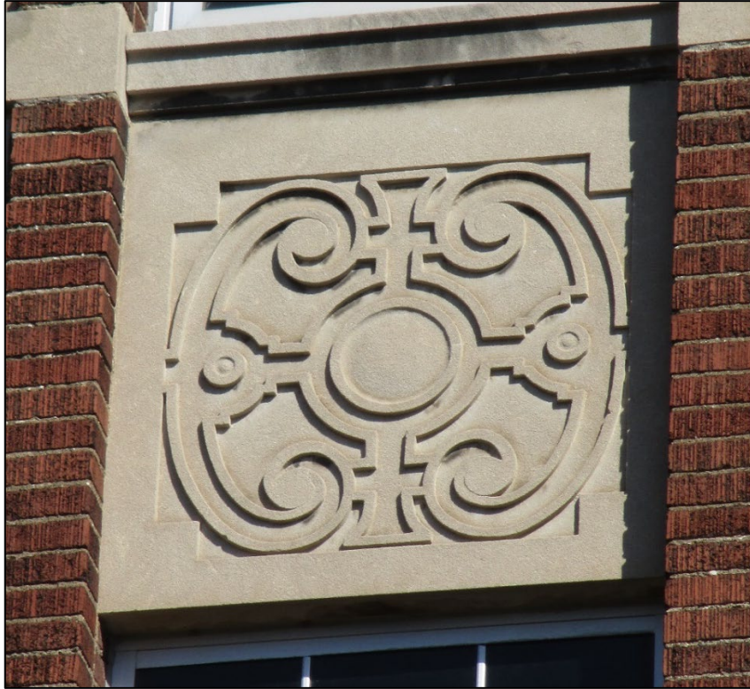
Figure 7: Detail view of stone decorative element.
