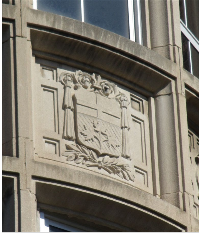
Figure 9: Province of Ontario coat of arms.
