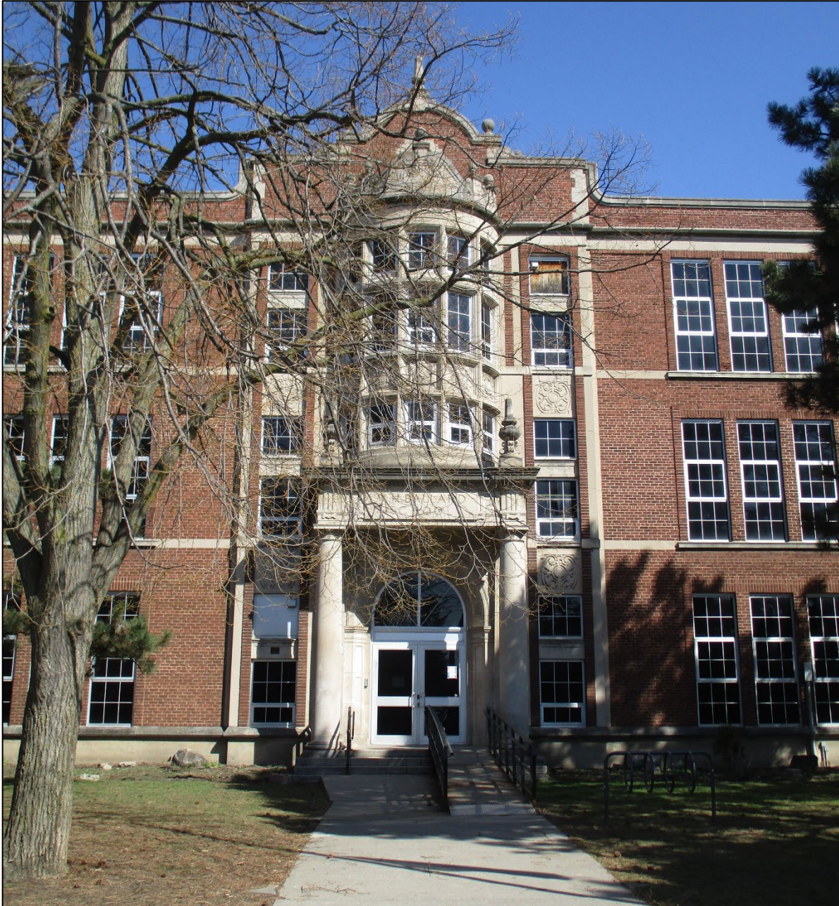
Figure 1: W.H. Ballard School, central front (south) elevation.
