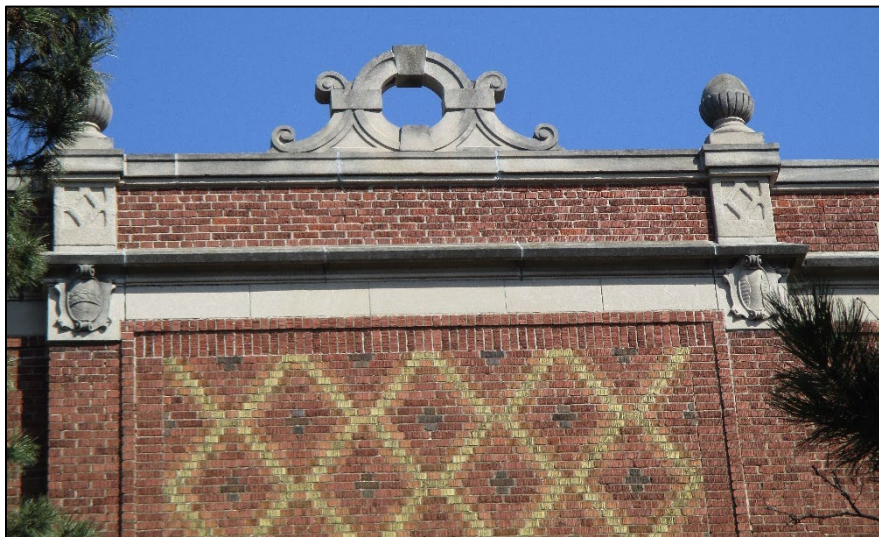
Figure 14: Detail view of decorative stone elements atop brick parapet.
