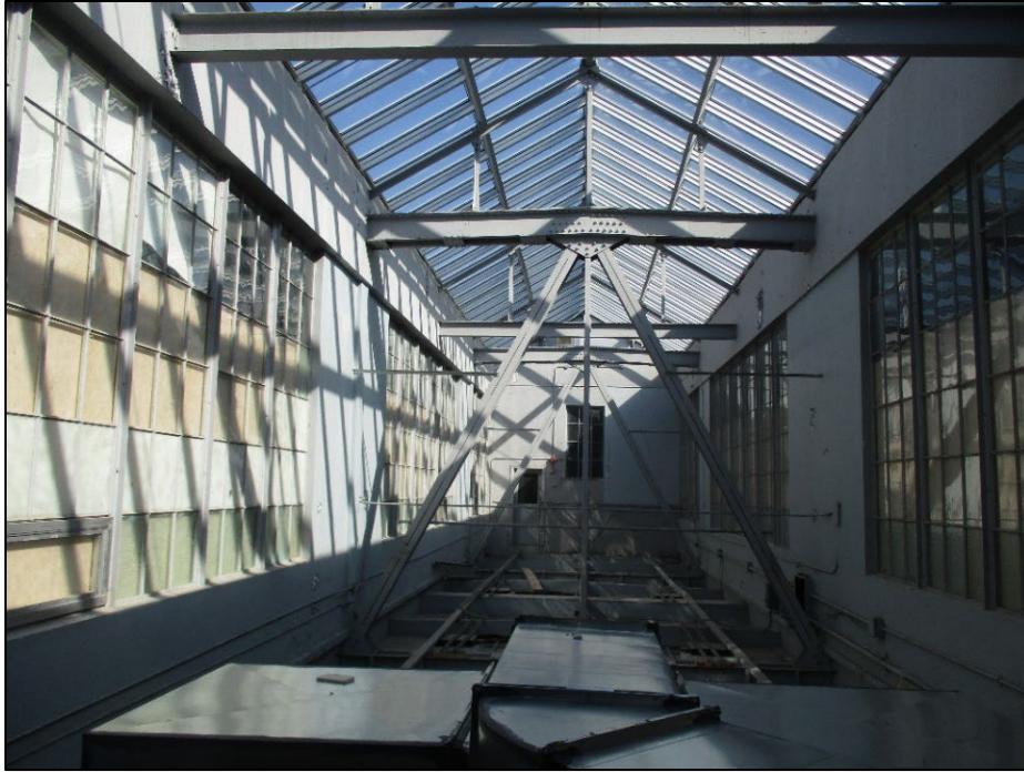
Figure 24: Covered light well and steel trusses supporting third storey classrooms.
