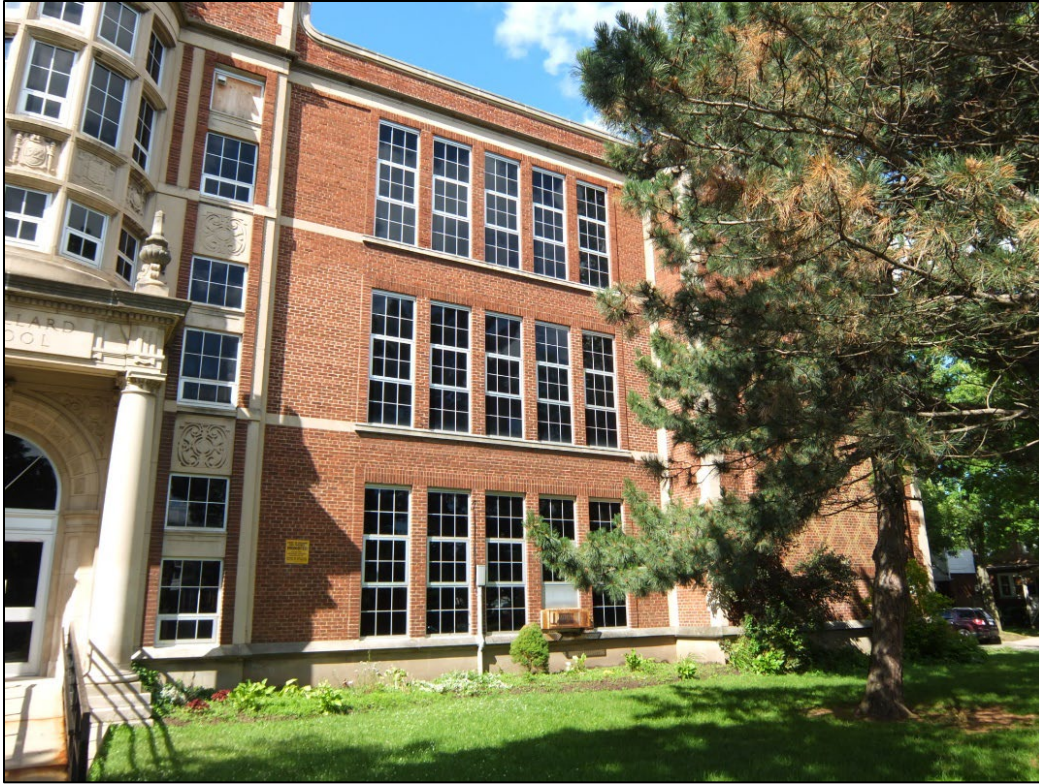
Figure 2: East side of south elevation. City of Hamilton staff, July 9, 2014.
