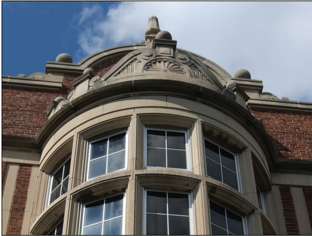
Figure 11: Detail view of parapet on circular bay. City of Hamilton staff, July 9, 2014.
