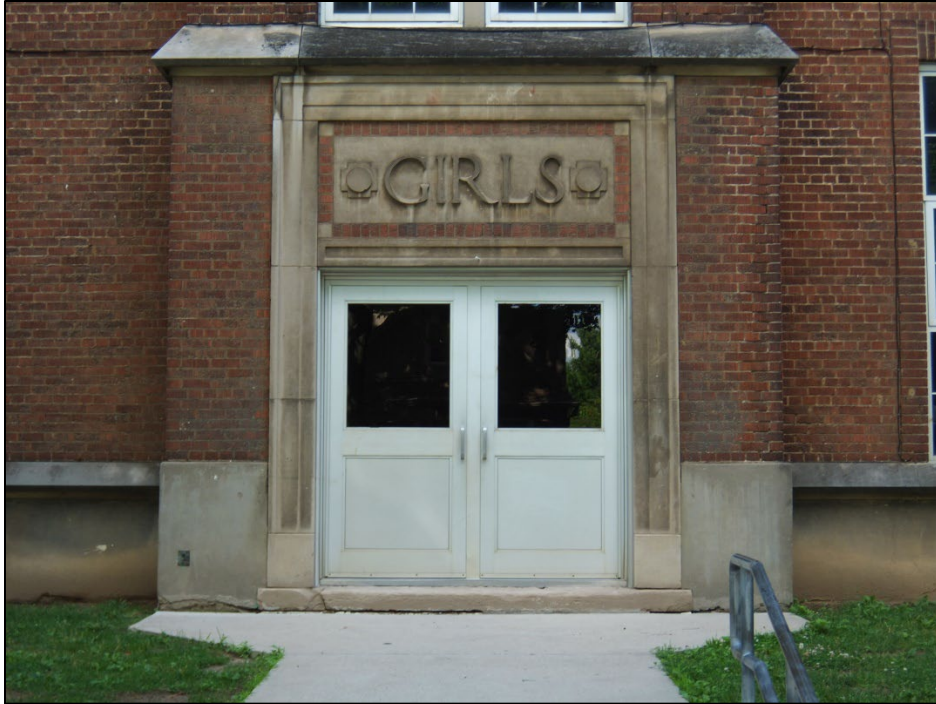
Figure 16: Detail view of entryway. City of Hamilton staff, July 9, 2014.
