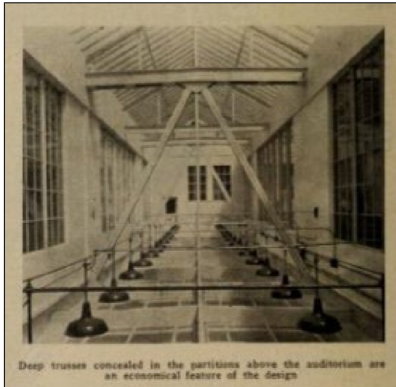
Figure 23: Covered light well and steel trusses supporting third storey classrooms, 1924 ( Contract Record and Engineering Review , December 1924)
