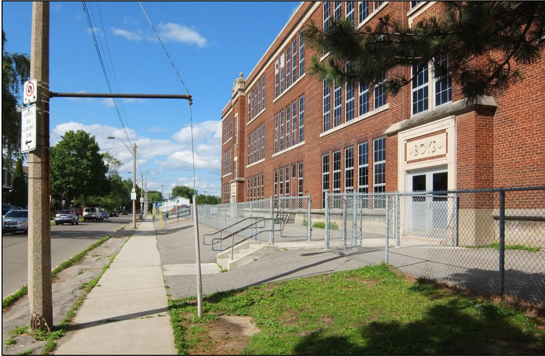
Figure 4: West elevation of subject property. City of Hamilton staff, July 9, 2014.
