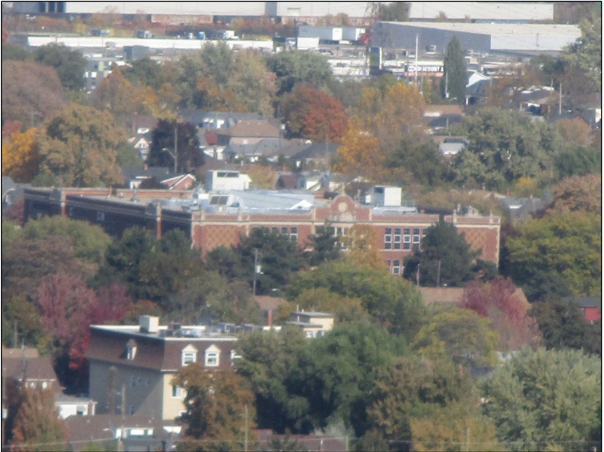
Figure 18: Contextual shot of subject property looking northeast from the mountain (City of Hamilton staff, October 22, 2024).
