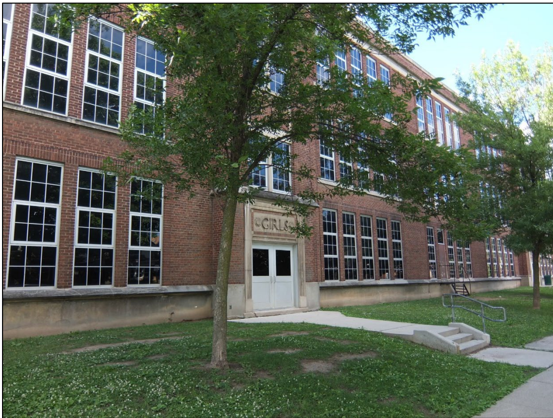
Figure 5: East elevation of subject property. City of Hamilton staff, July 9, 2014.
