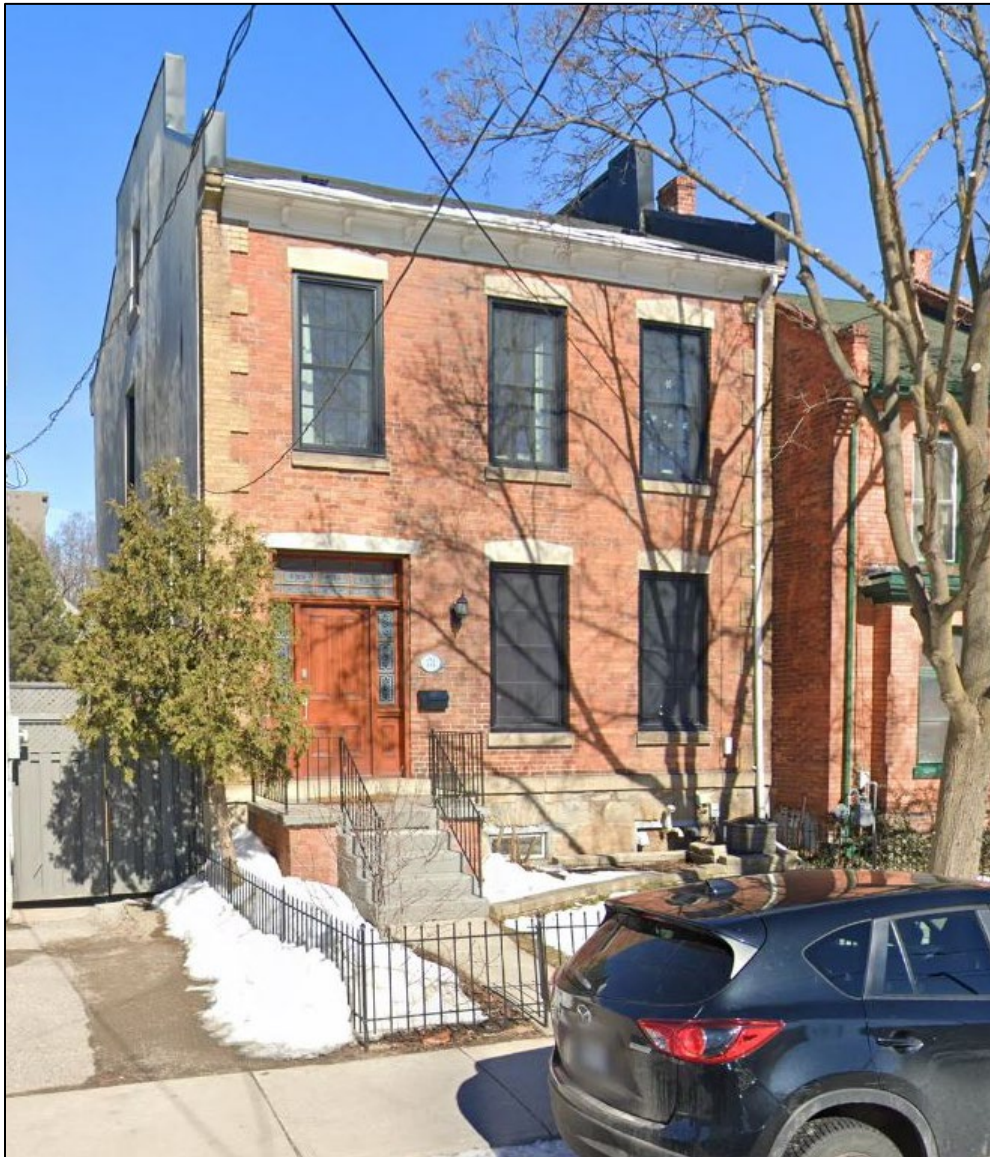
Figure 1: View of 171 Forest Avenue from the road.
