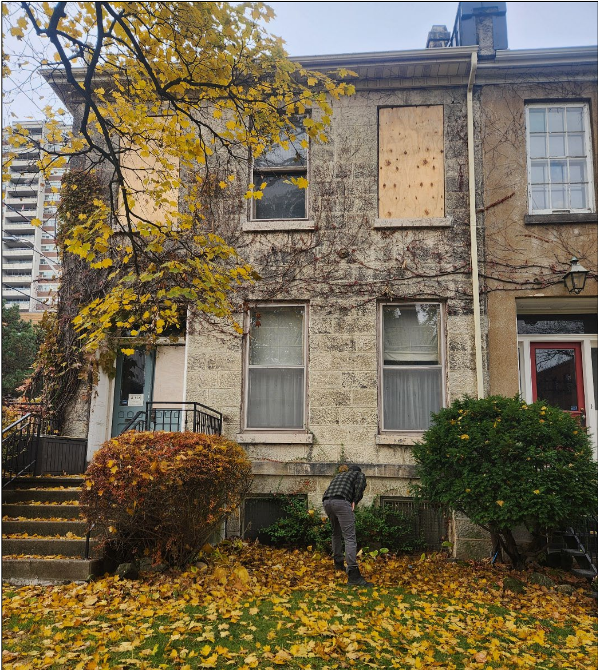
Figure 1: View of the MacNab façade showing existing conditions.
