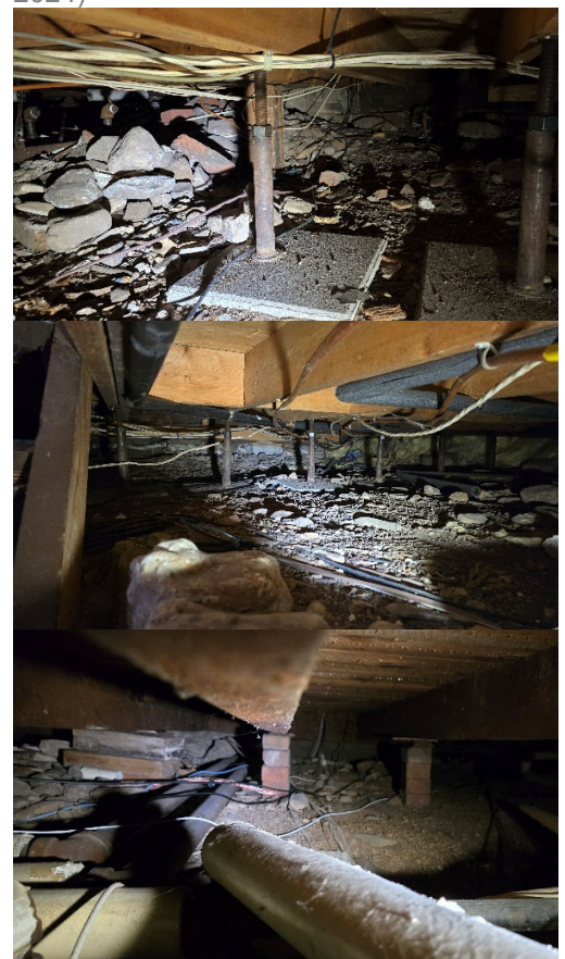
Basement & crawl space (Owner, 2024)
