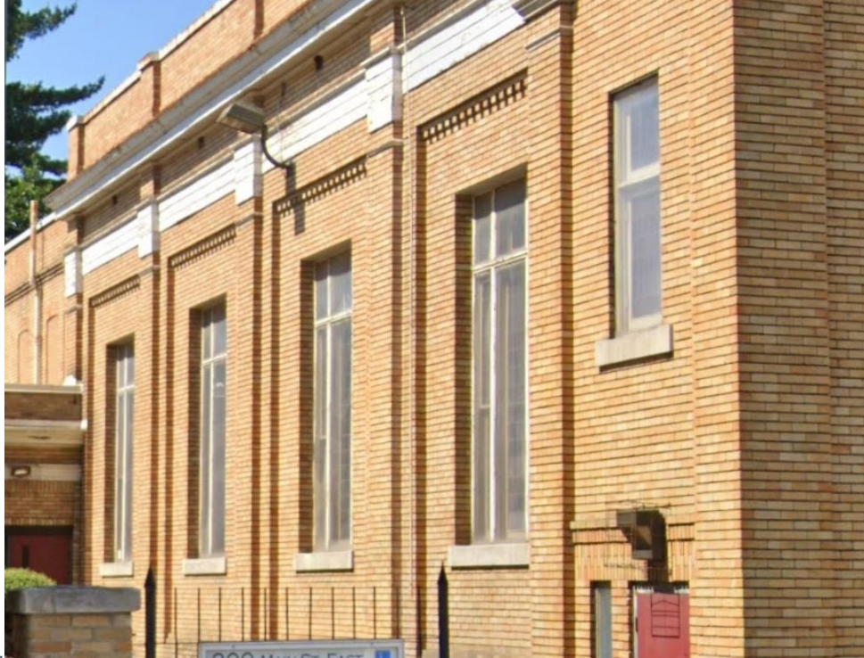
Figure 11: Detail view of side (east) elevation. Google Earth, January 2025.
