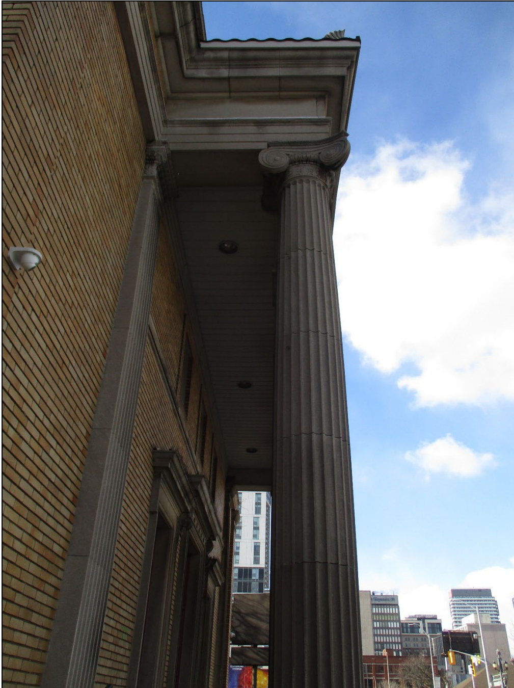
Figure 2: Detail view of front (north) elevation.
