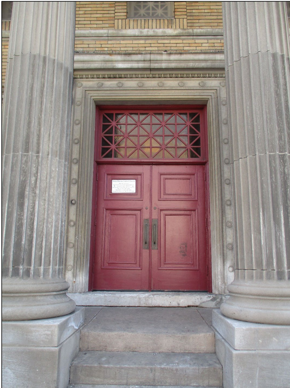
Figure 3: Detail view of main entrance on front (north) elevation.
