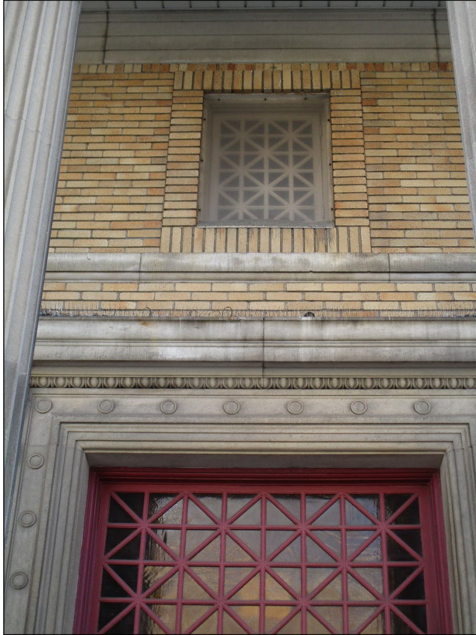
Figure 5: Detail view of windows.
