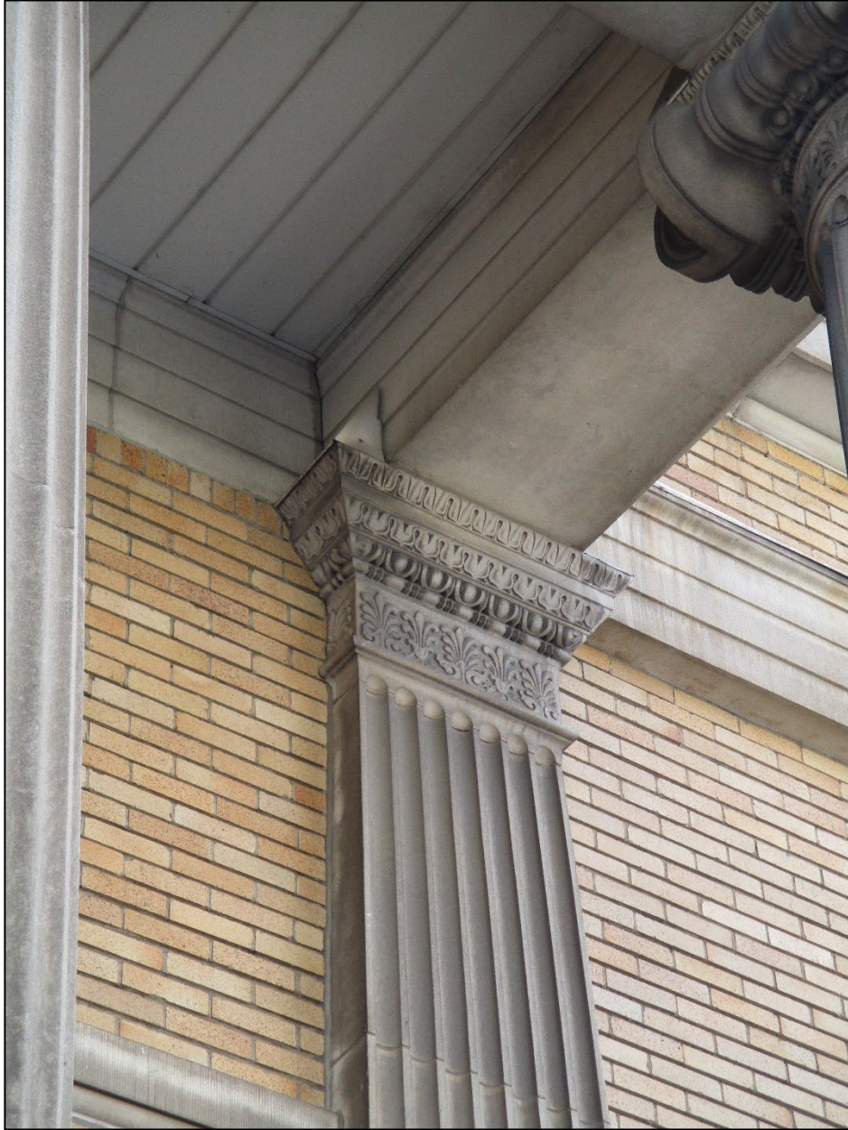
Figure 7: Detail view of pilaster.
