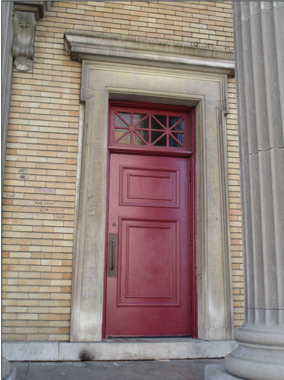
Figure 6: Detail view of secondary entrance on front (north) elevation.
