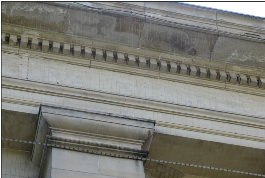
Image 5: Close-up of the dentilated cornice (July 10, 2012)
