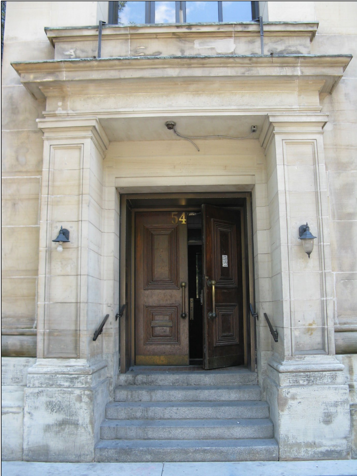
Image 7: Close-up of the recessed central entrance with stone surround, flanking columns with moulded panels and Doric capitals and entablature (July 10, 2012)
