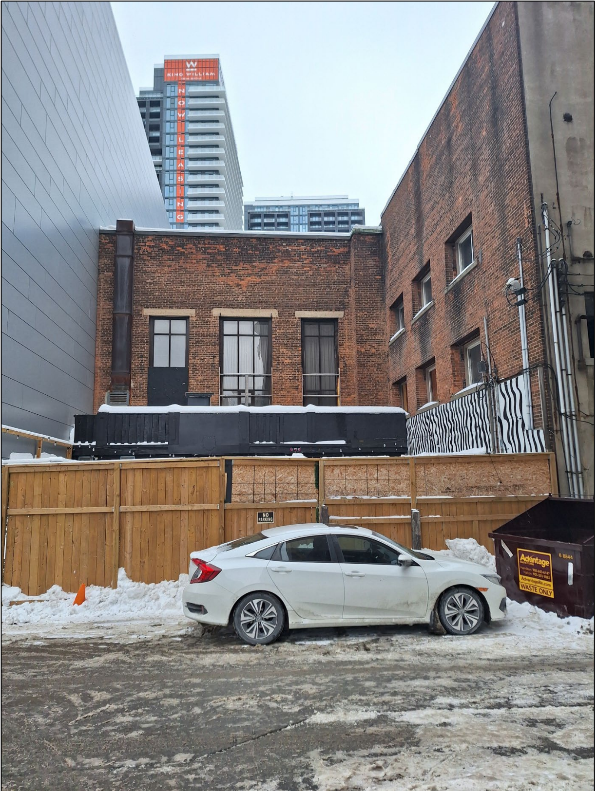
Image 8: Rear (south) elevation (Feb 21, 2025)
