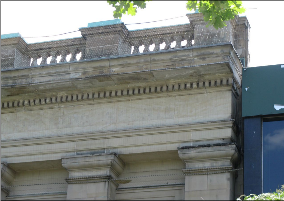
Image 4: Close-up of the stone balustrade, entablature, and doric capitals (July 10, 2012)
