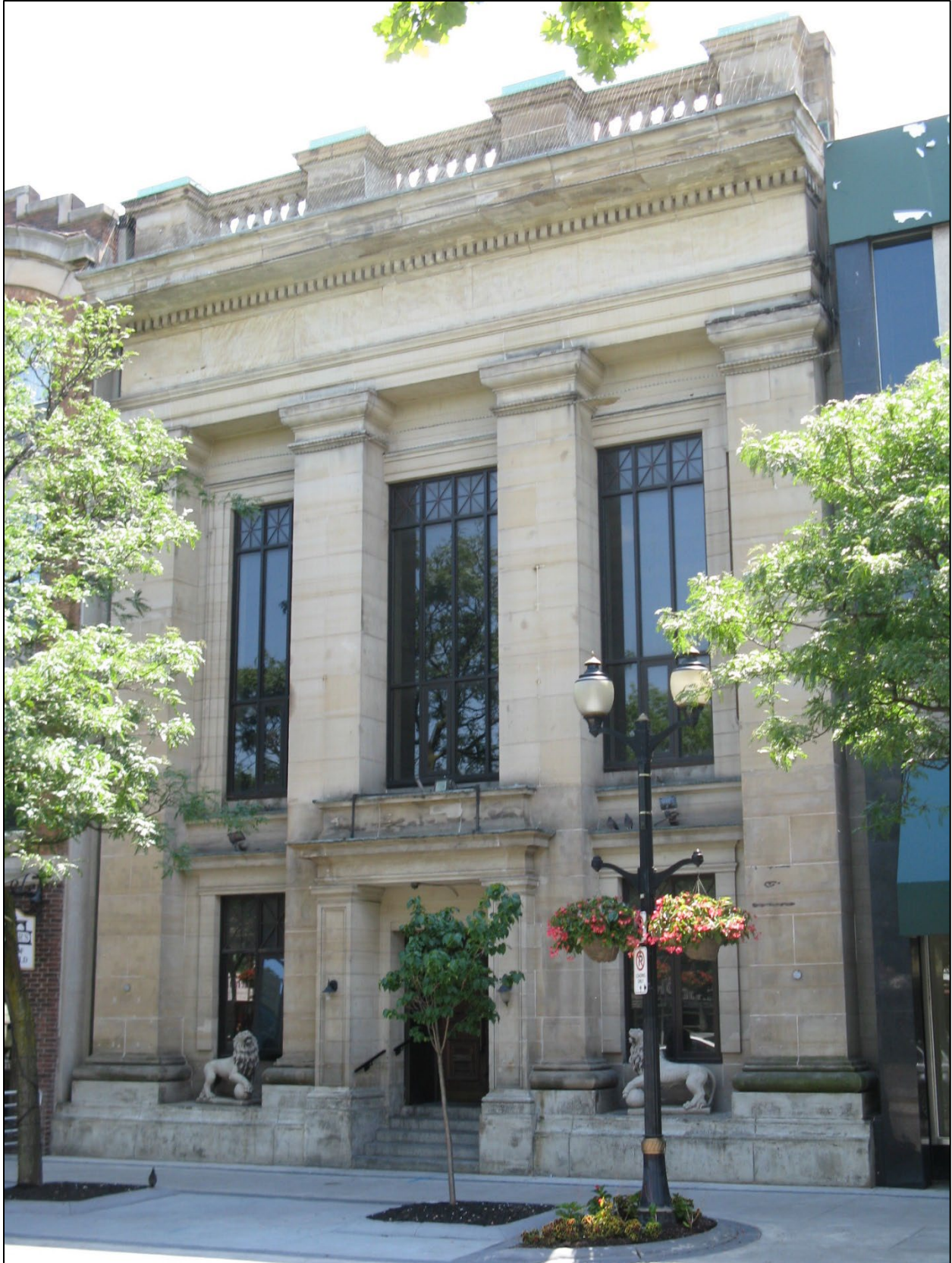
Image 3: Front (north) elevation (July 10, 2012)
