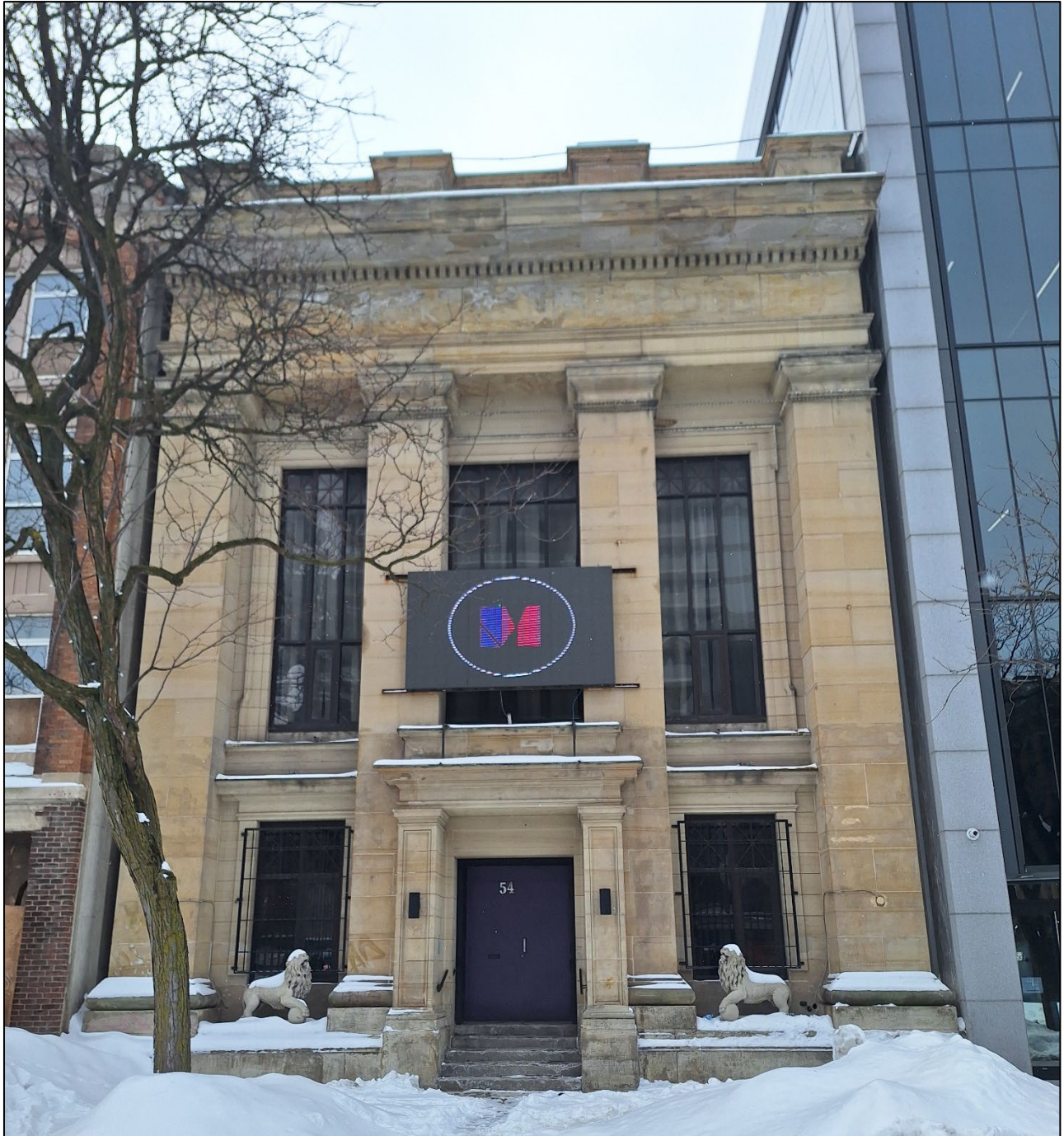
Image 1: Front (north) elevation (February 21, 2025)
