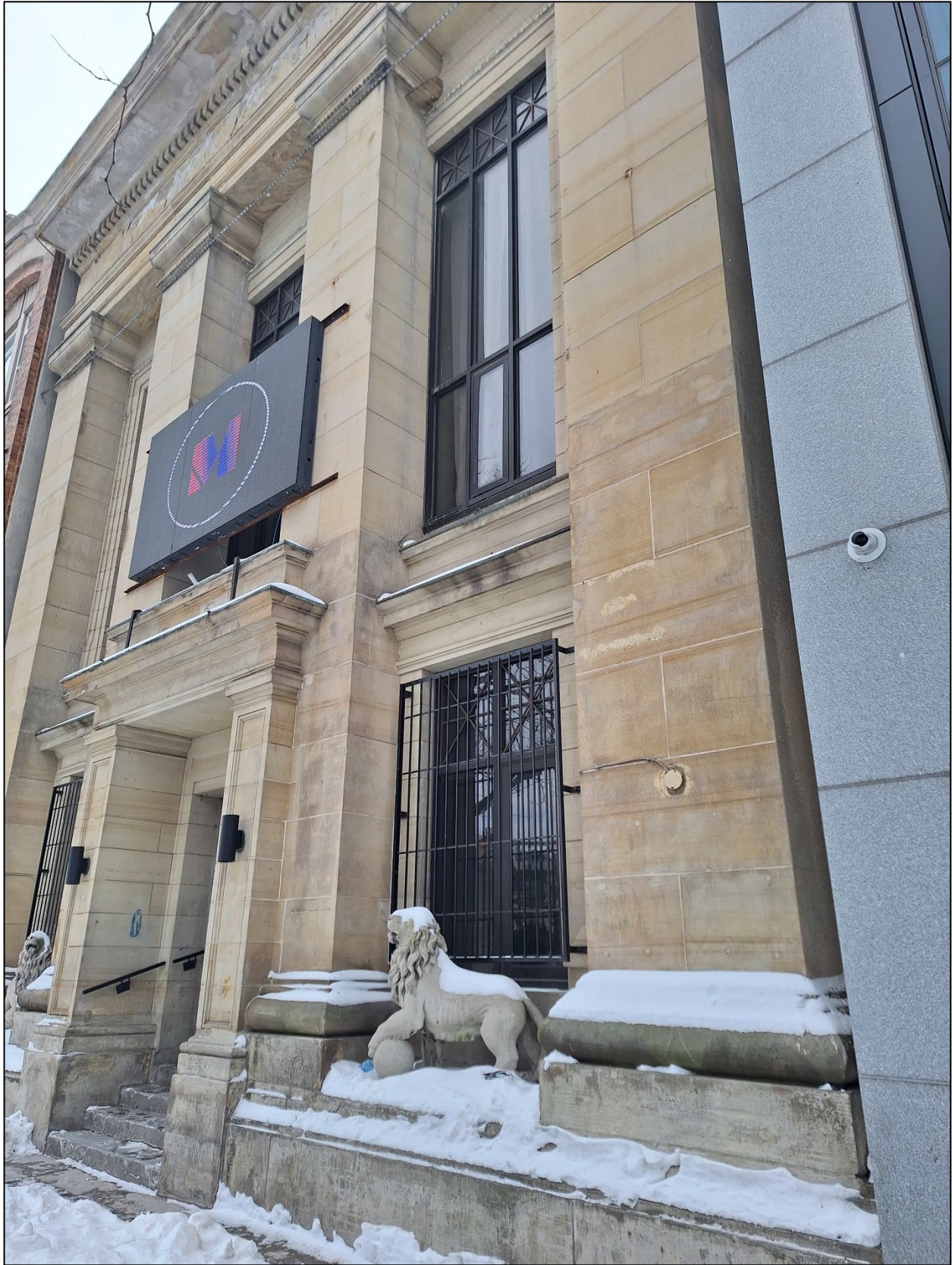
Image 2: Front (north) elevation (February 21, 2025)
