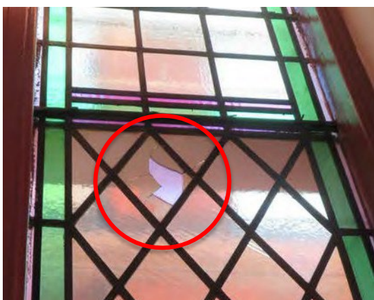
Church Interior – damaged 1908 stained-glass windows in the east (left) and west (right) side elevations
