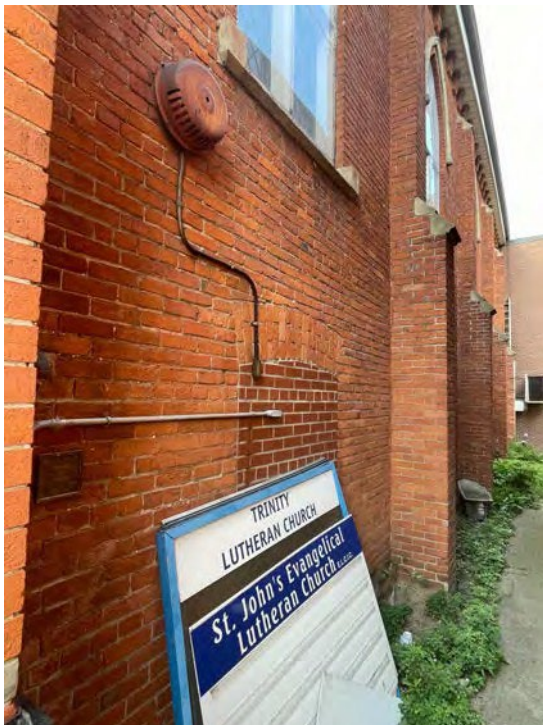
East wall of the Church – basement window infilled
