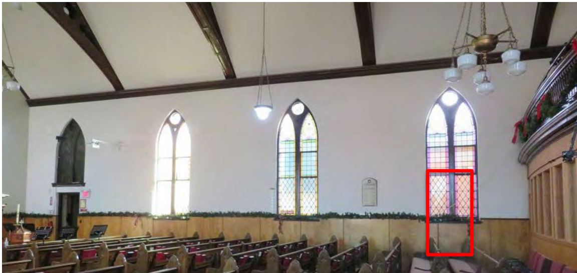
East wall of the Church – the stained-glass window in Bay 2 must be modified for a doorway into the proposed addition.
