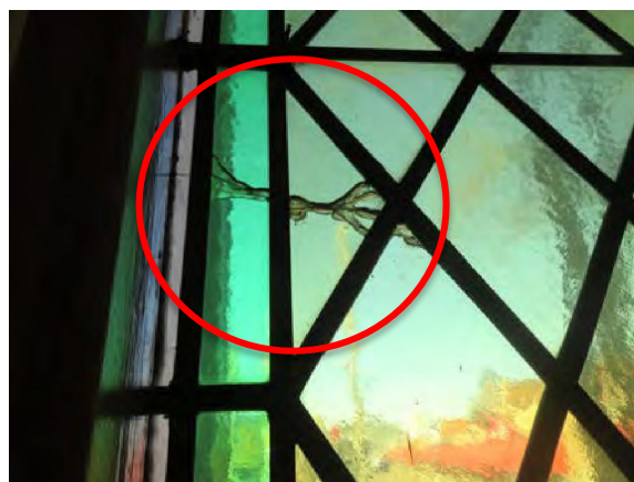
Church Interior – damaged 1908 stained-glass windows in the east (left) and west (right) side elevations
