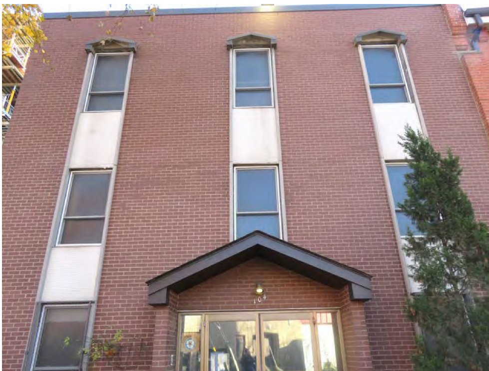
1969 Sunday School Addition that replaced the attached 1867 Parsonage – the original windows have been replaced – cladding has been installed on top of the concrete window caps and above the door – the trim framing the window bays is Queenston limestone
