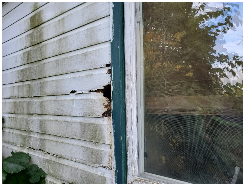
Photo No 06: Rotted Siding
