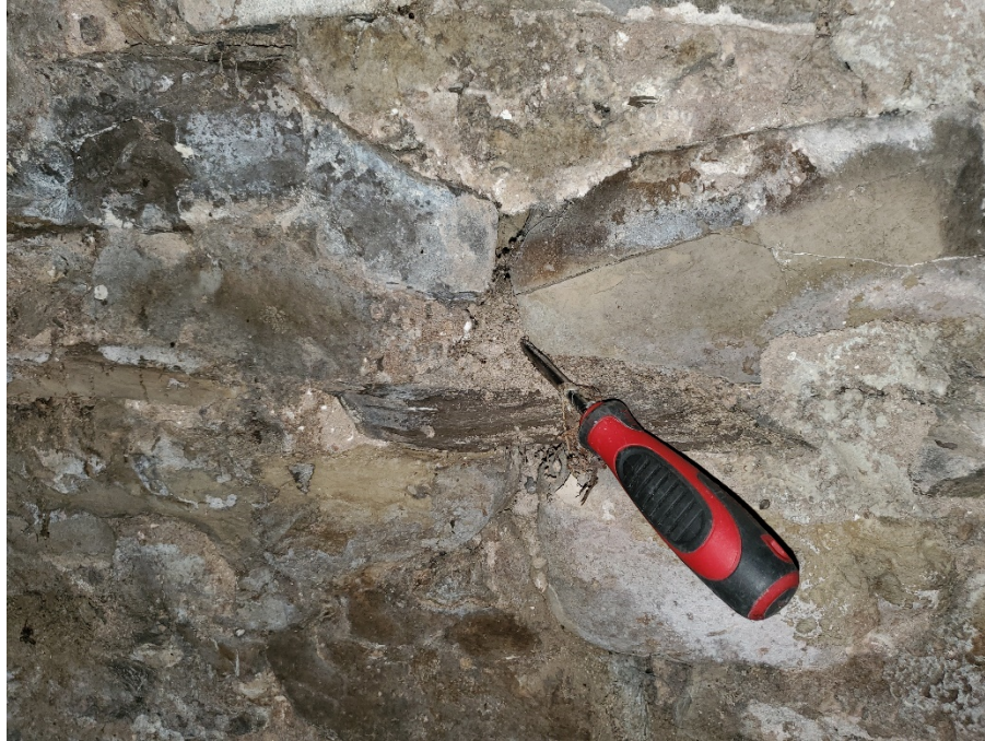
Photo No 11: Spalled Mortar Joint
