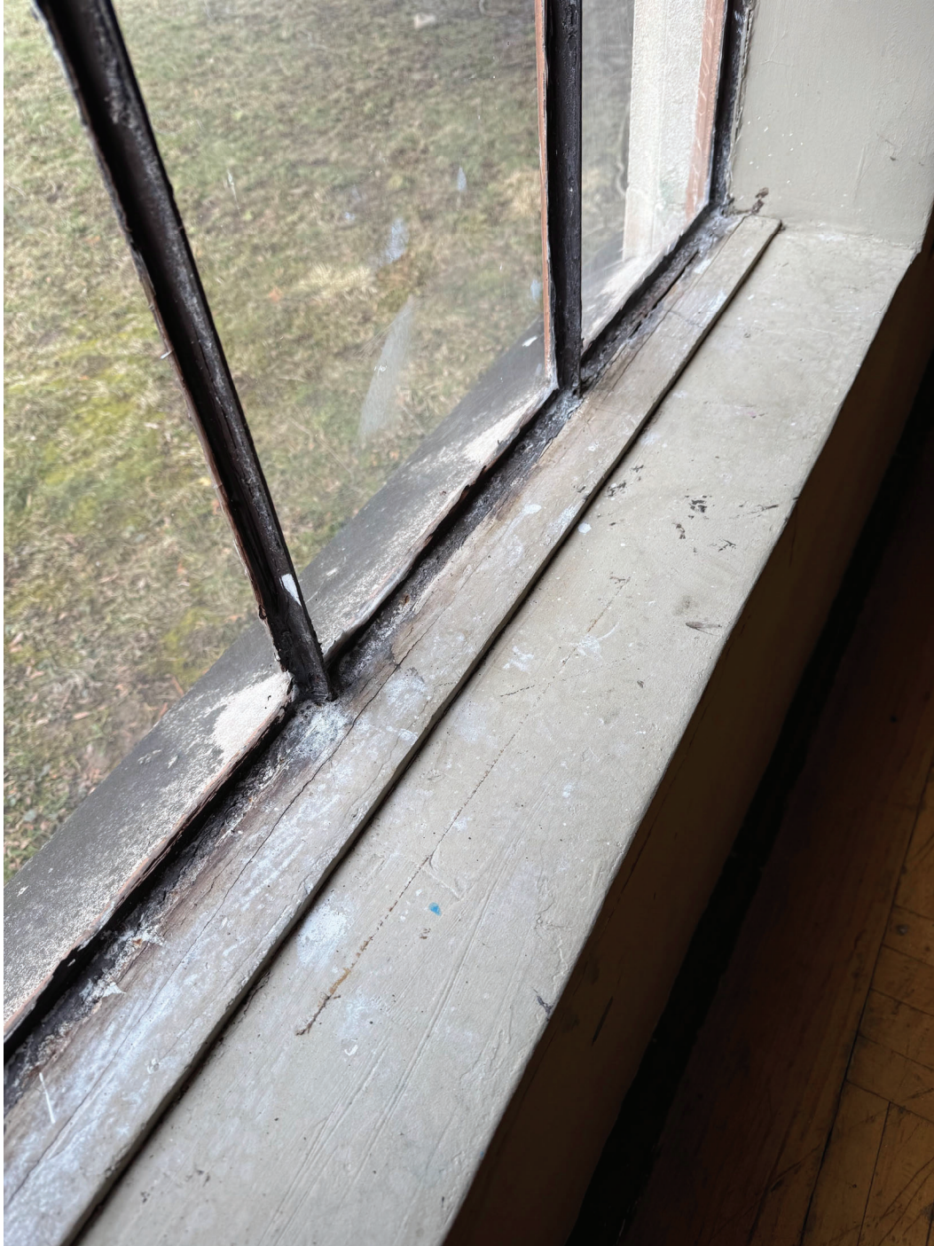
Figure 1 – Existing corroded steel window frame
