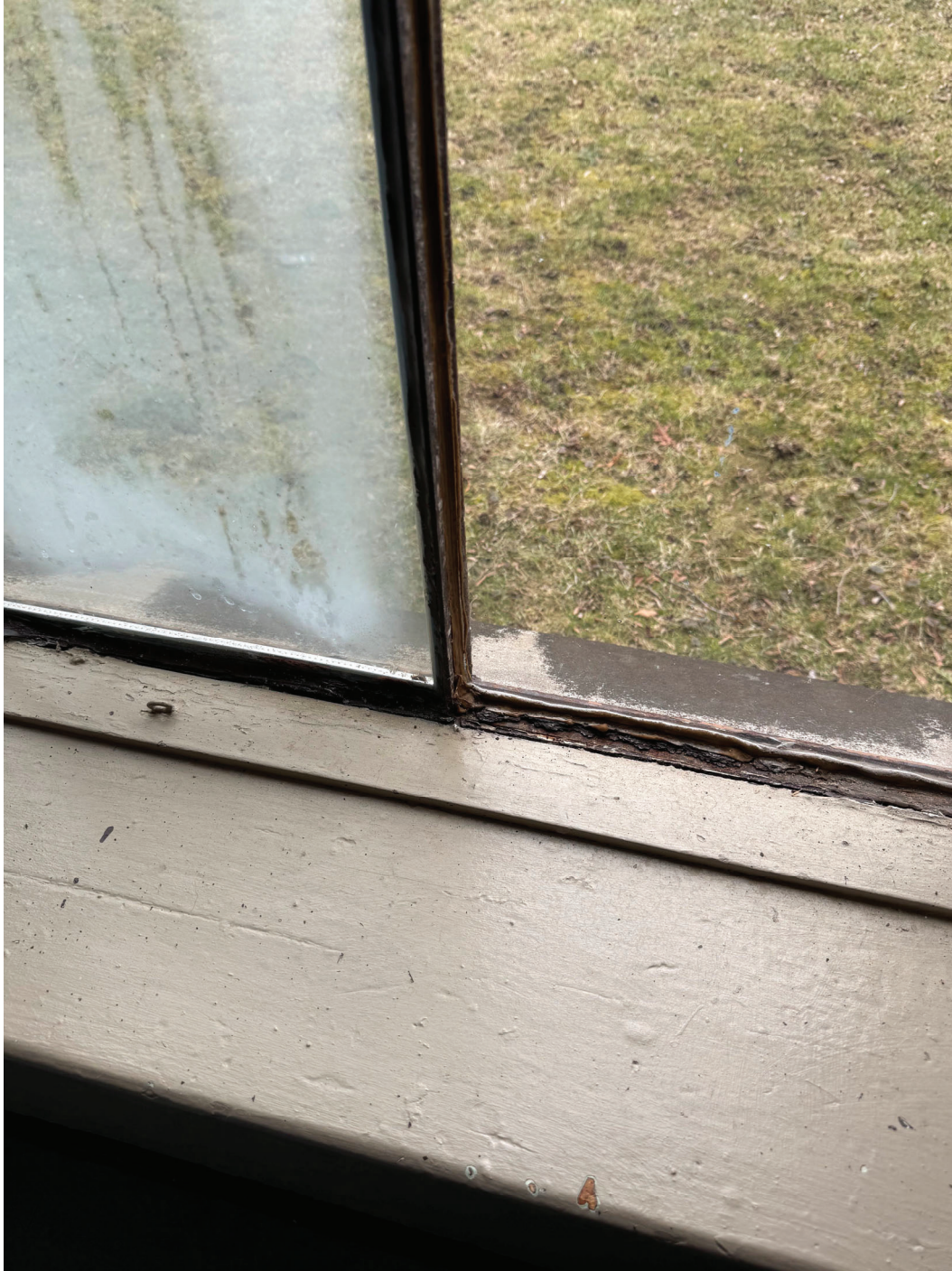
Figure 5 – Existing corroded steel window frame.
