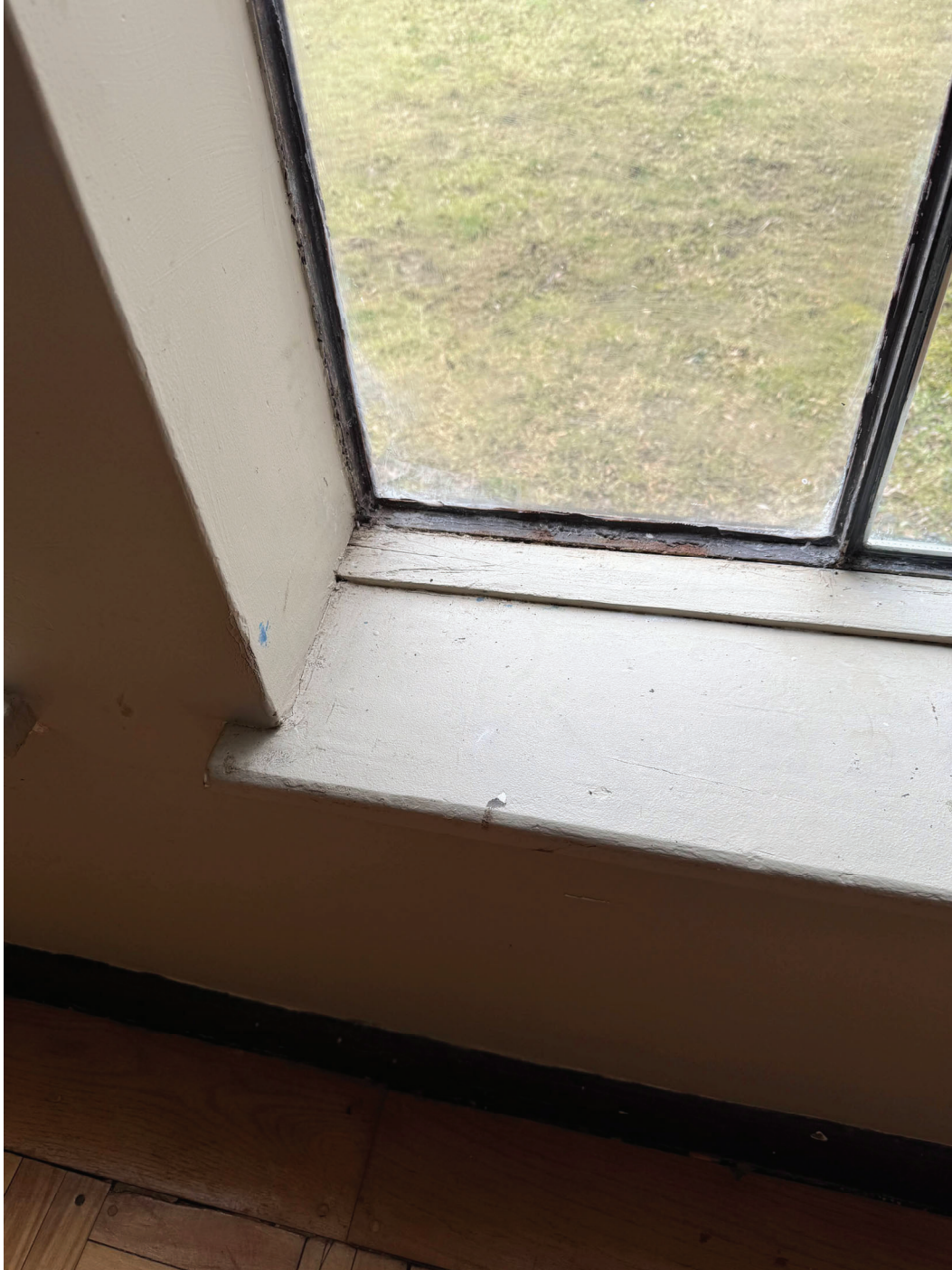
Figure 2 – Existing rusted steel window frame
