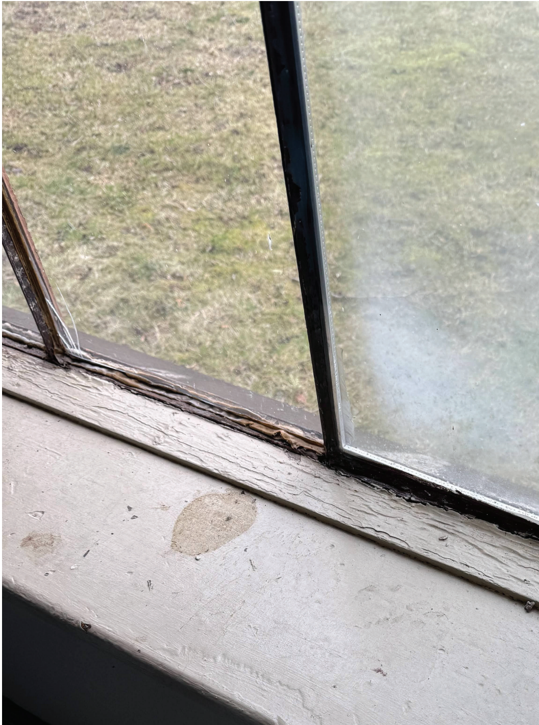
Figure 6 – Existing corroded steel window frame with cracked glass, and water damaged wood window sill.
