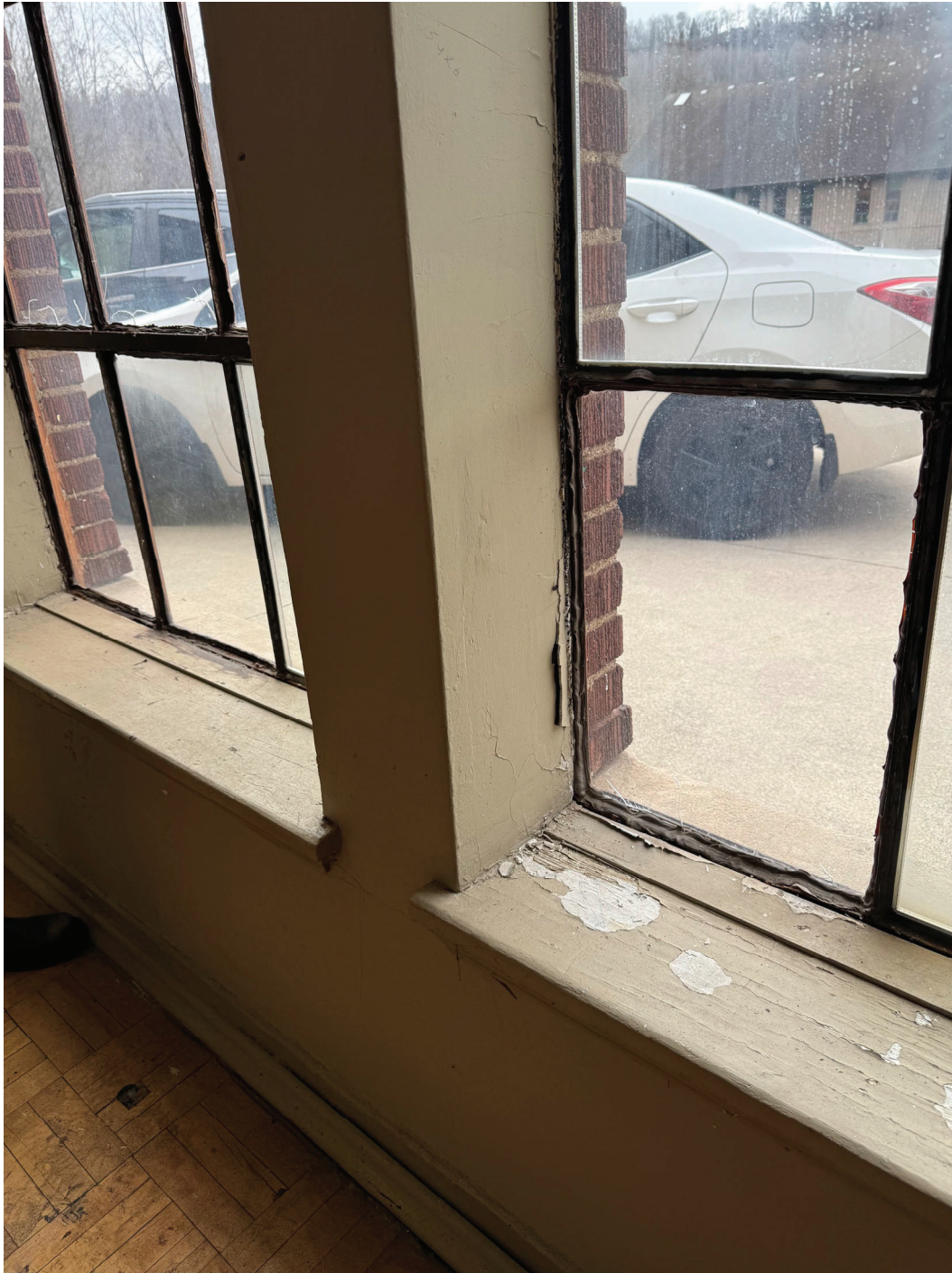
Figure 4 – Existing corroded steel window frame patched with caulking, and water damaged wood window sill.
