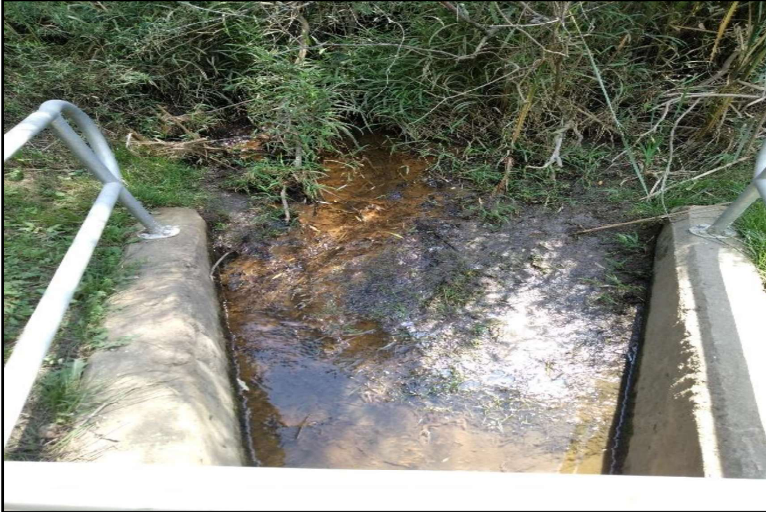
Photograph 3. Flows entering the culvert at the downstream end of the off-site stormwater pond. Photo taken on September 5, 2025, facing west.
